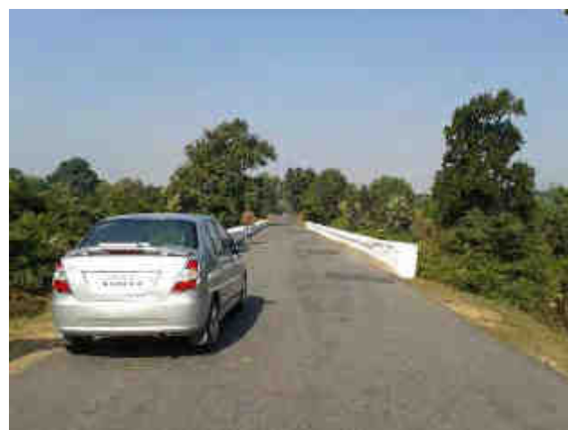
Unprotected approach to bridge with high embankment, Km 6+100
