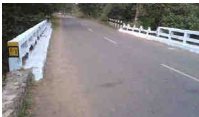
Parapets of Culvert/Bridge not delineated, Km 8+500 and Km 11+700
