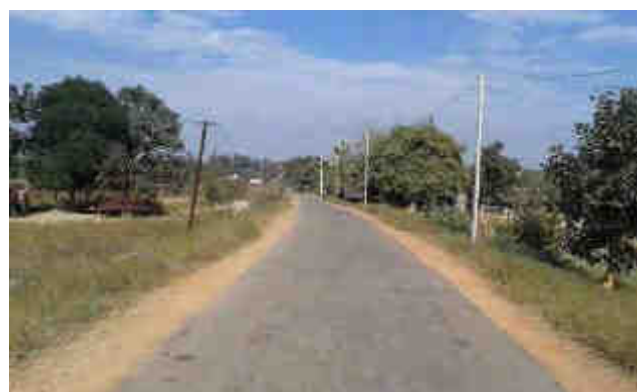
Lack of delineation on the entire stretch of road. Photographs of stretches (i) Km 6+000 to 7+000, and (ii) Km 4+000 to 5+000
