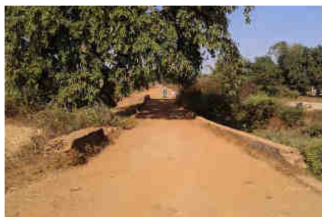
Parapets of Culvert/ Bridge not delineated, Km 0+500 and Km 4+500
