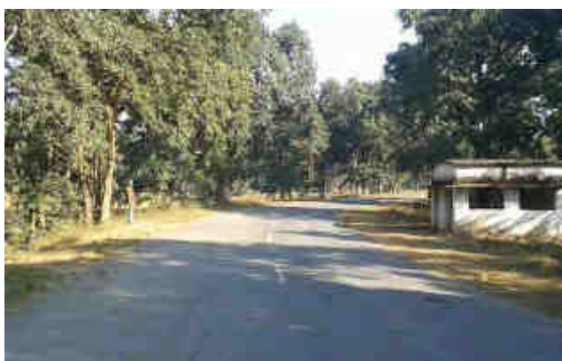
Sharp curve with restricted visibility due to building, Km 3+800
