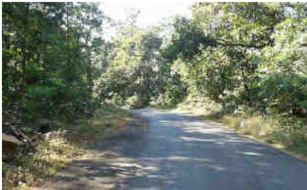
Sharp curve with restricted visibility in forest/ghat section at Km 174+900
