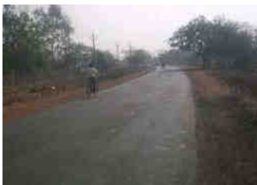
Curve at Km 6+500
