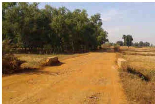
Parapets of Culvert/ Bridge not delineated, Km 0+500 and Km 4+500
