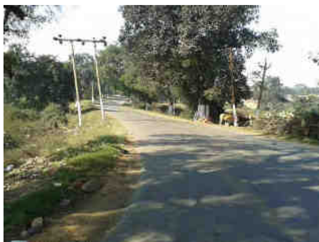
Trees and poles very near to road edge Km 3+000 to Km 4+000
