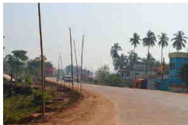
Curve at Km 8+600
