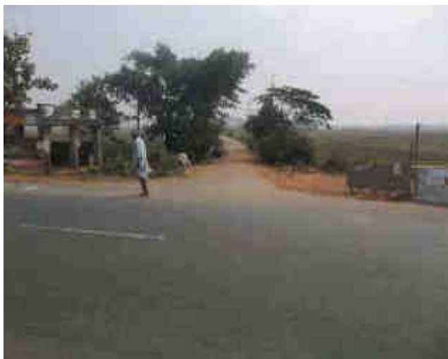
Side road with poor visibility due to vegetation at Km 225+200
