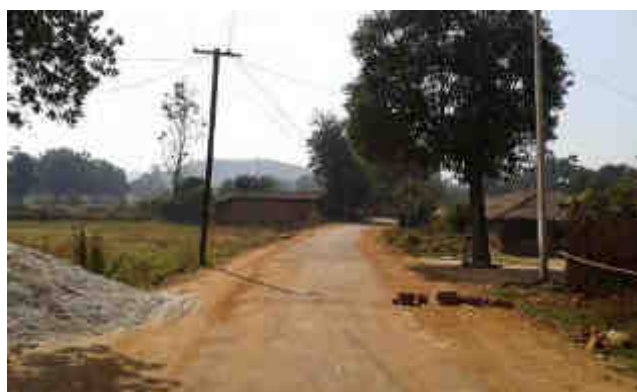
Lack of delineation on the entire stretch of road. Photographs of stretches (i) Km 6+000 to 7+000, and (ii) Km 4+000 to 5+000
