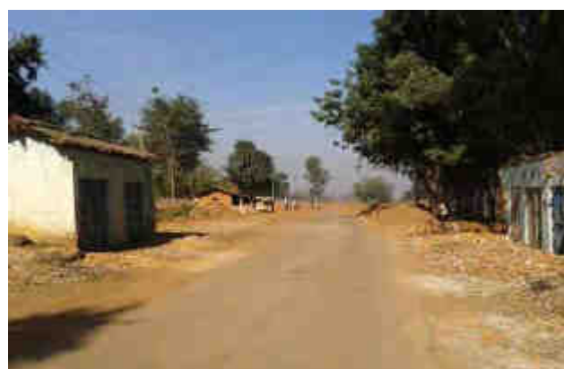
Lack of center line and edge line in the stretch from Km 12+000 to 13+000
