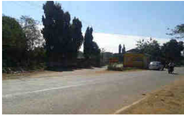
Km 314+600, intersection of NH-49 with Kuchinda town road (north of Kuchinda)
