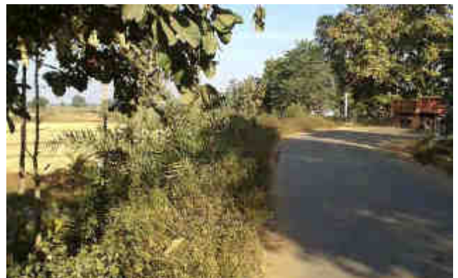
Sharp curve on high embankment without edge protection near railway crossing at Bamra (Km 198+700)
