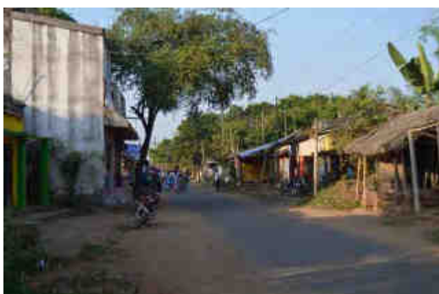
Built up area at Km 4+200
