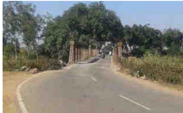
Parapets of bridge not delineated, Km 313+300 and Km 317+400
