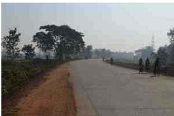
Curve at Km 4+400
