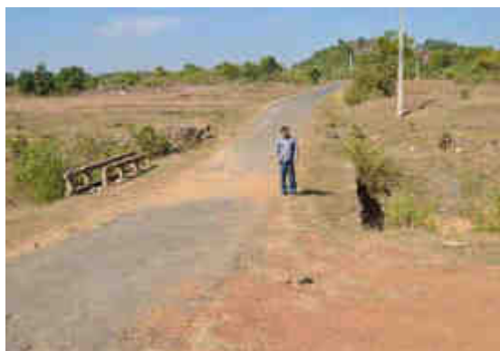
Absence of protection and OHM on structure at Km 7+400 and Km 10+300
