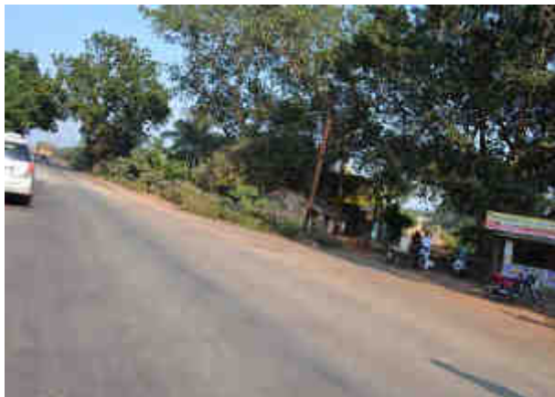
Skewed Side Road at Km 5+800
