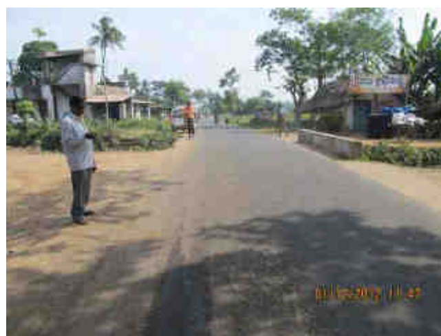
absence of parapet wall at Km 24+800
