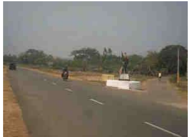
Skewed side road at Km 30+100
