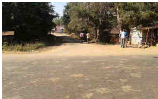
Restricted visibility from access road due to buildings and trees on corners, Km 312+900
