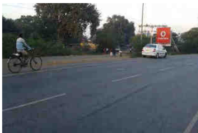
Side Road joining SH-10 at acute angle, Km 149+800
