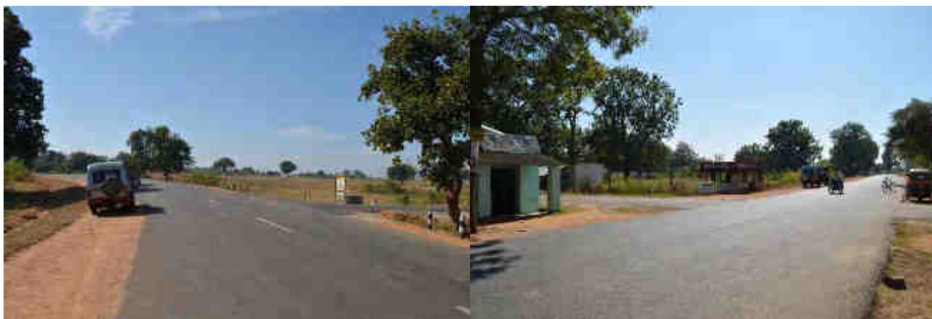
Minor Junctions at Km 66+950 and at Km 76+800
