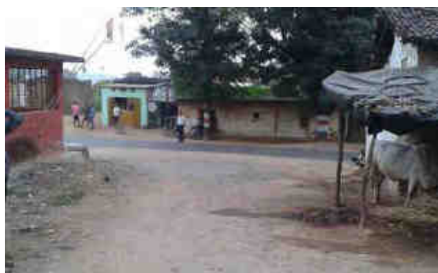
Restricted visibility from access road due to buildings on corners, Km 6+500
