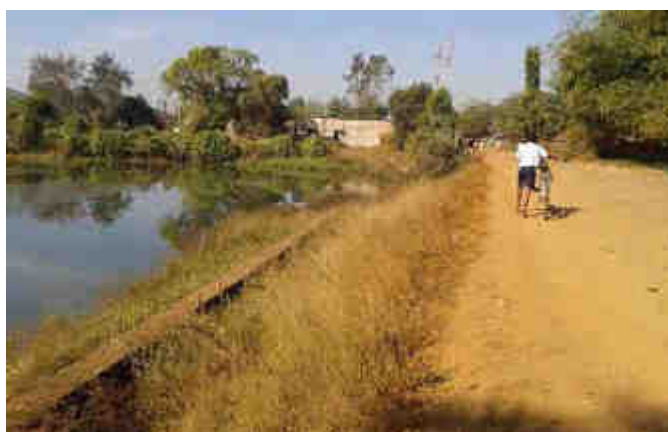
Pond near the road without delineation or any edge protection, Km 2+200
