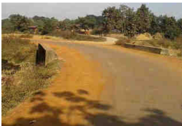
Parapets of Culvert/Bridge not delineated, Km 6+200 and Km 0+600
