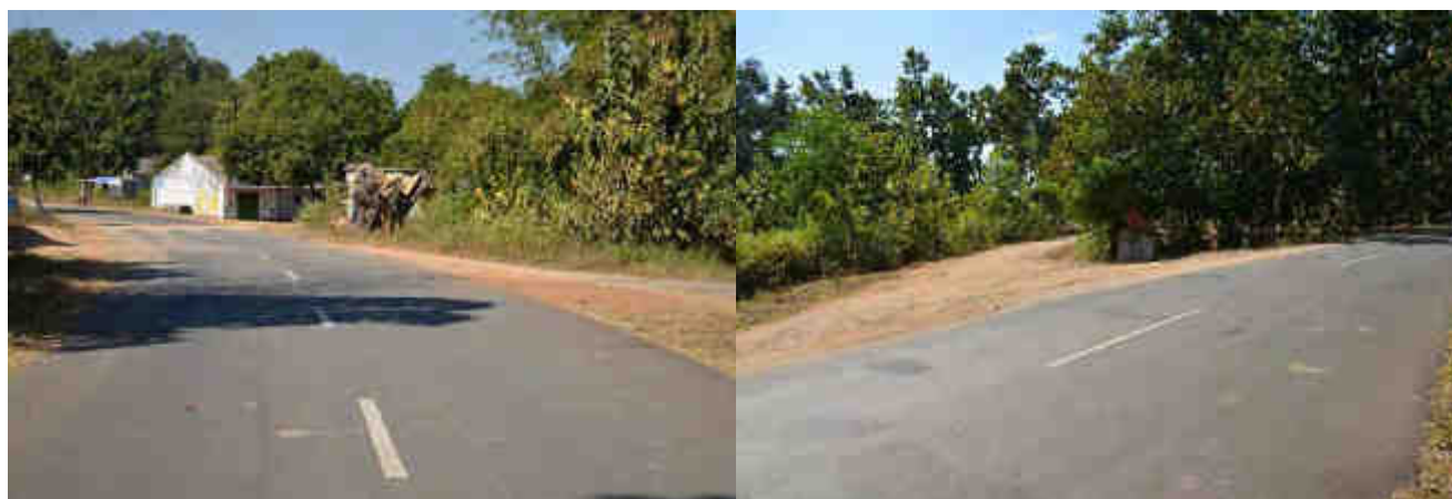
Skewed Side Road at Km 42+900 and Km 45+800
