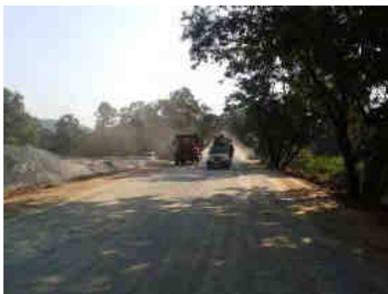
Road construction Km 35+000 to 36+000
