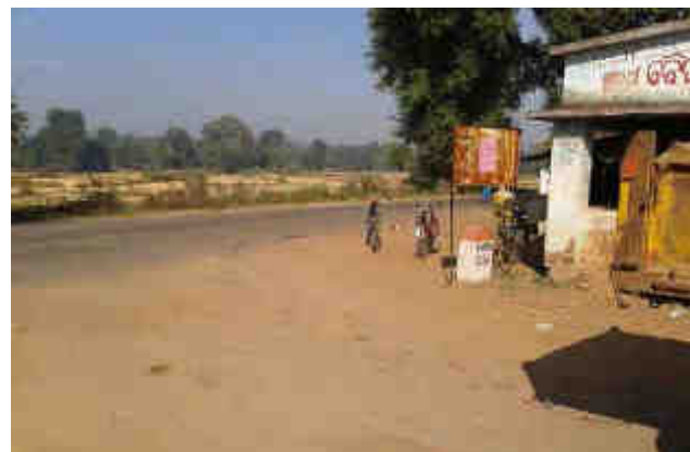
Side road joining at Km 7+100 – visibility restricted due to buildings on both the corners(view from side road)
