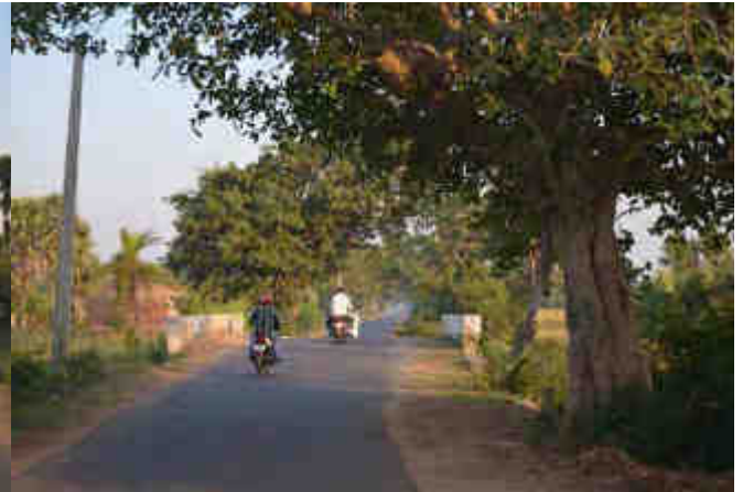
Culvert at Km 10+000
