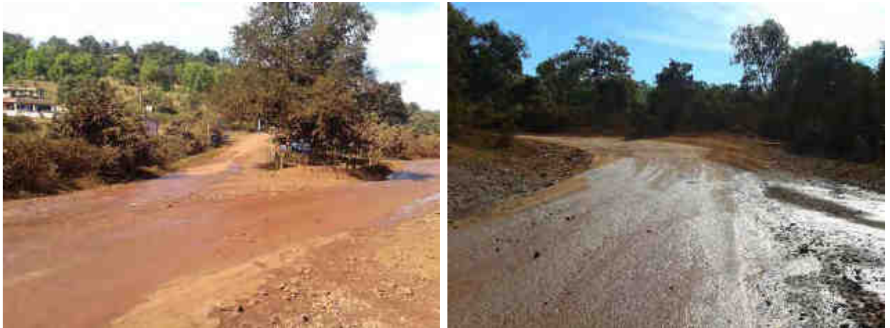
Km 13+600, Intersection of ODR with road from SAIL mines – trees in the central island and approach to intersection descending from the hairpin bend
