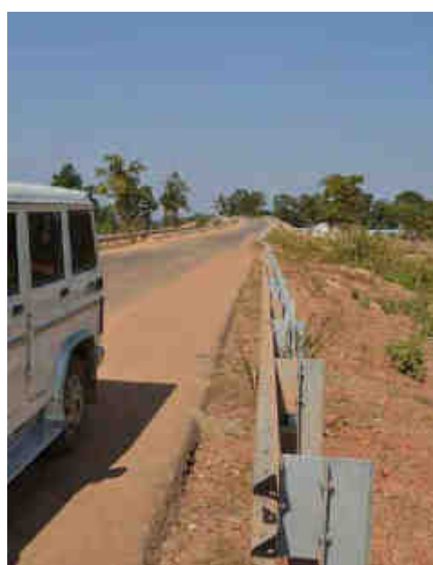
Crash Barrier very near to pavement edge
