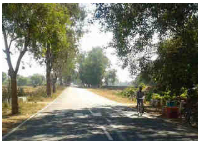
Trees very near the road edge, Km 319-320
