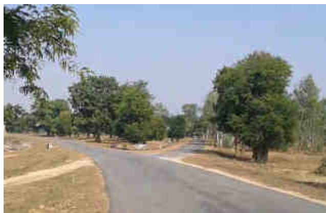
Side road joining at skew angle Km 21+000
