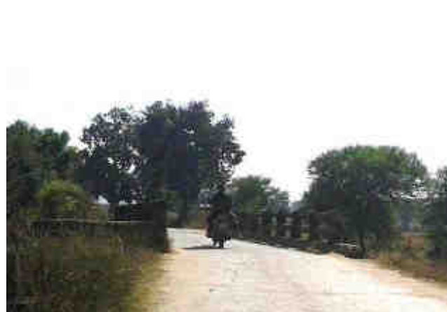
Parapets of Culvert/Bridge not delineated, Km 6+200 and Km 0+600
