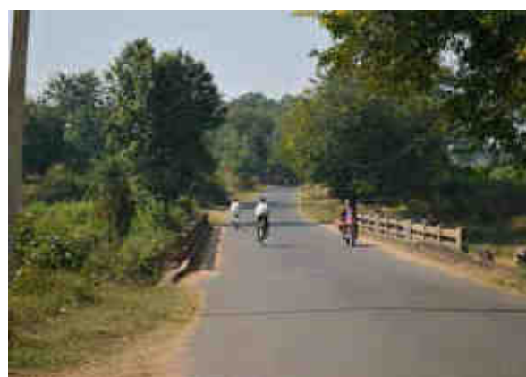
Minor Bridge at Km 48+700
