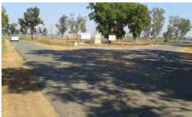
Side road joining at skew angle Km 157+400
