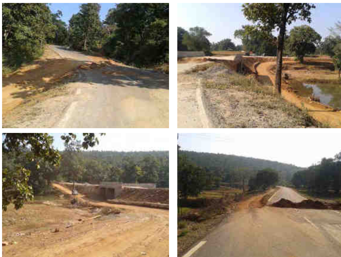
Km 31+800 – Traffic diversion at the site of construction of culvert
