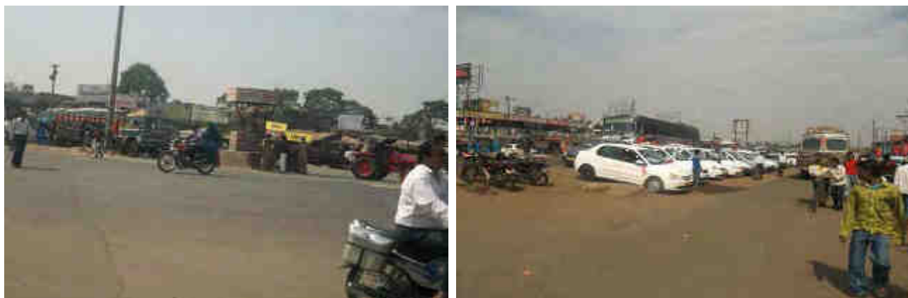
Poor junction layout and on street parking at roundabout at Km 219+000
