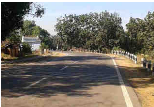
Sharp curve at Km 39+900
