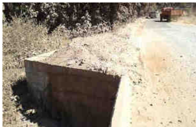
Unprotected approaches to the causeway, Km 24+000
