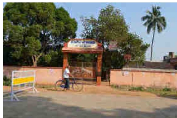
School at Km 8+400 in Biribati Village
