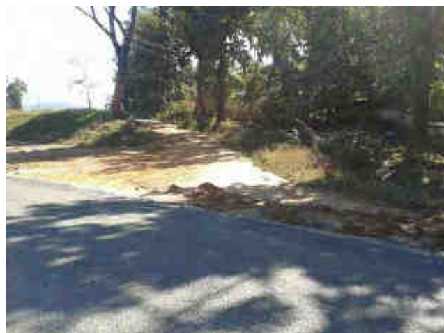
Side road joining at skew angle Km 24+350
