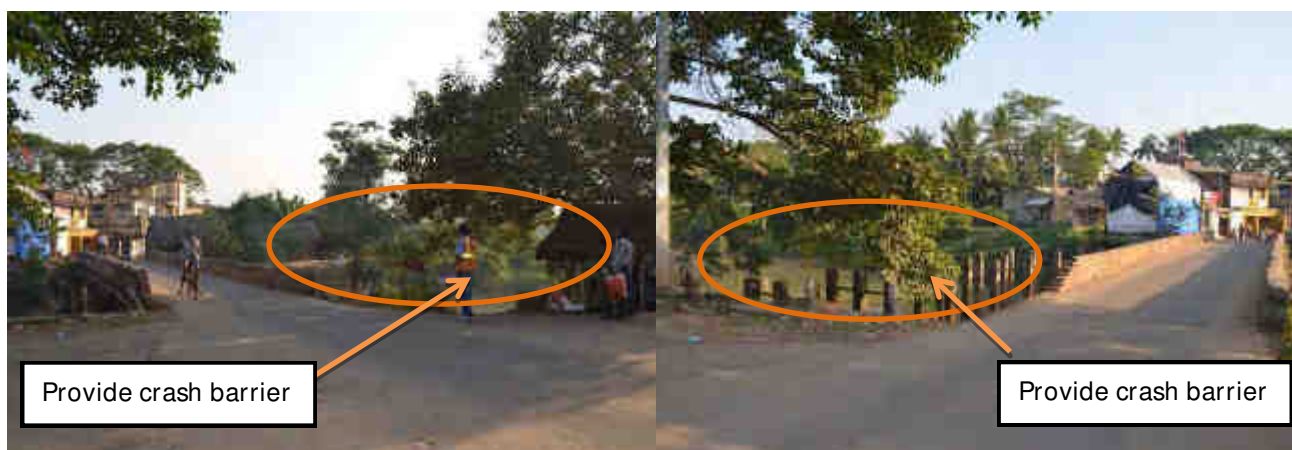
Junction at Km 4+950
