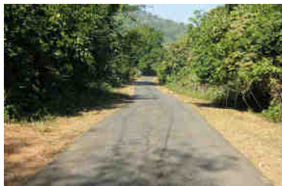
Road marking missing
