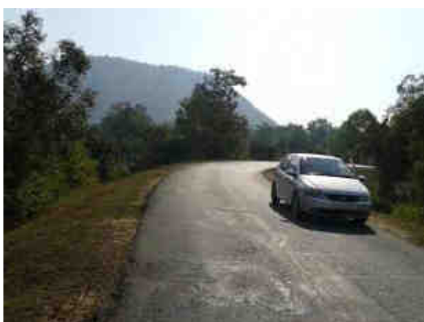
Unprotected approach to bridge with high embankment, Km 6+100
