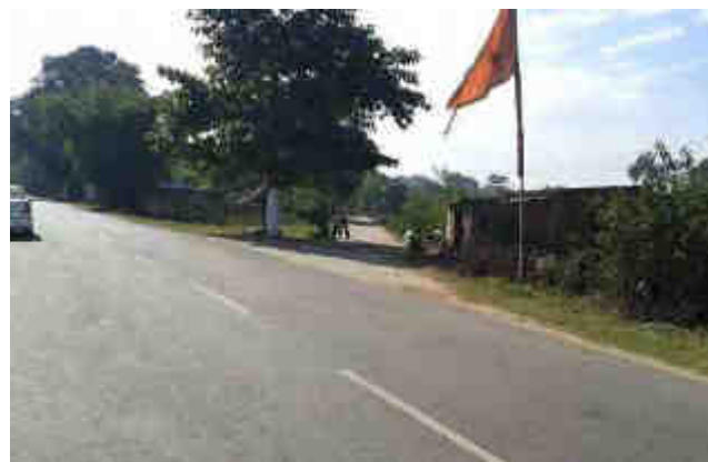
Side road joining at acute angle, Km 4+600
