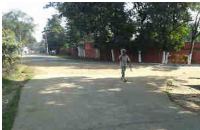
Side road joining on curve, Km 3+600 (view from side road)
