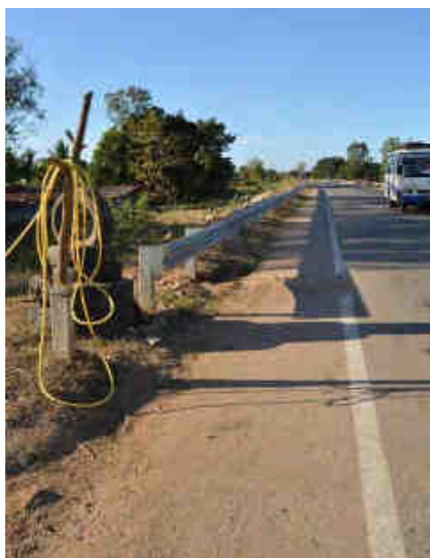
Crash Barrier very near to pavement edge
