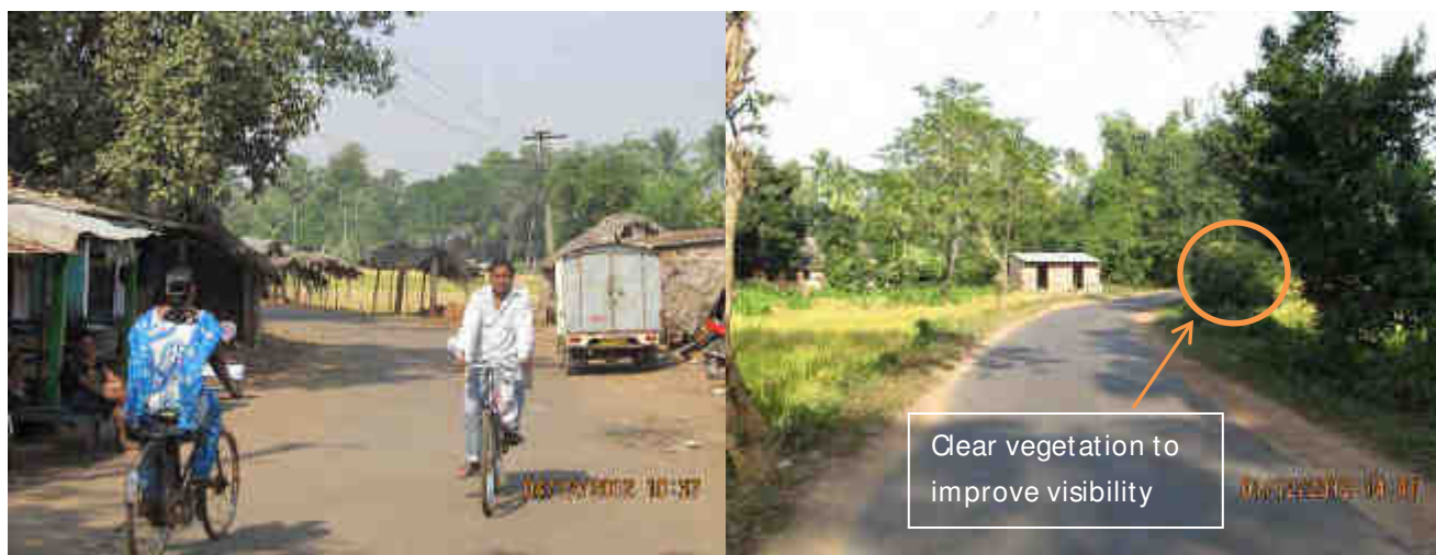
Sharp Curves on Project Road at Km 26+600 and Km 3+550
