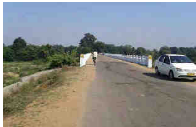
Bridge at Km 20+600, No protection on approaches
