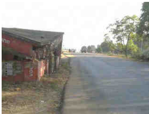
Building (LHS) and Tree (RHS) very near to the road edge, Km 60+000 to 61+000
