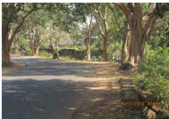
Broken Parapet wall at Km 13+600
