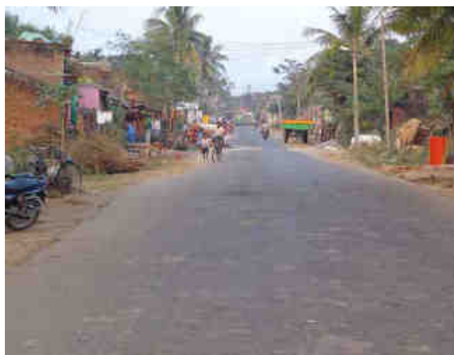
Km 39+000 (Chundangapur village)
