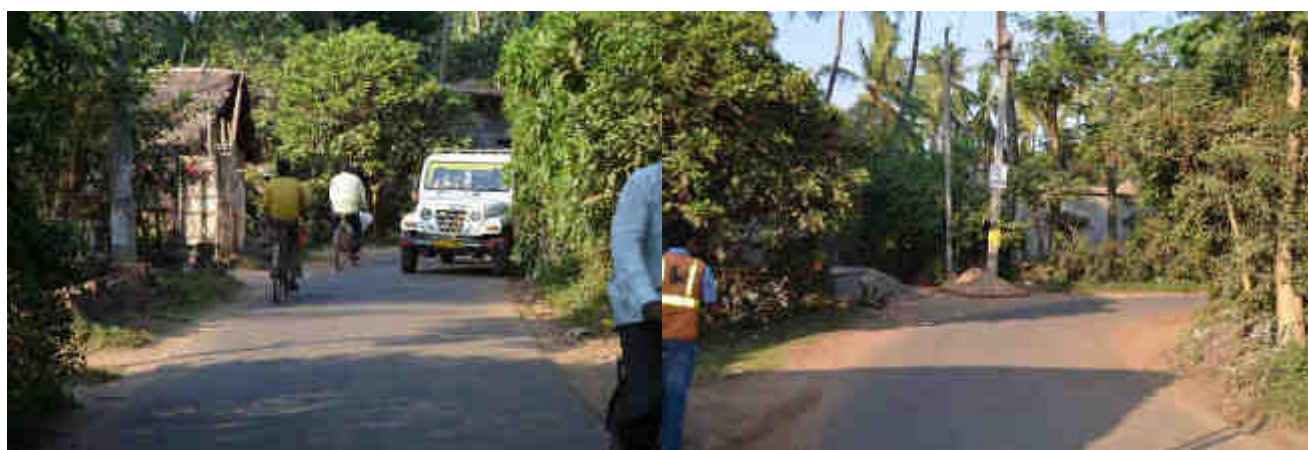
Sharp Curves on Project Road at 1+300 and 1+450
