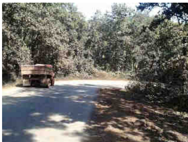
Hairpin bend with steep gradient at Km 22+100
