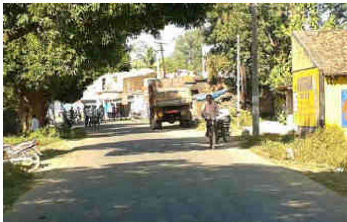
Poles very near the road edge in BUA, Km 169+000-169+700
