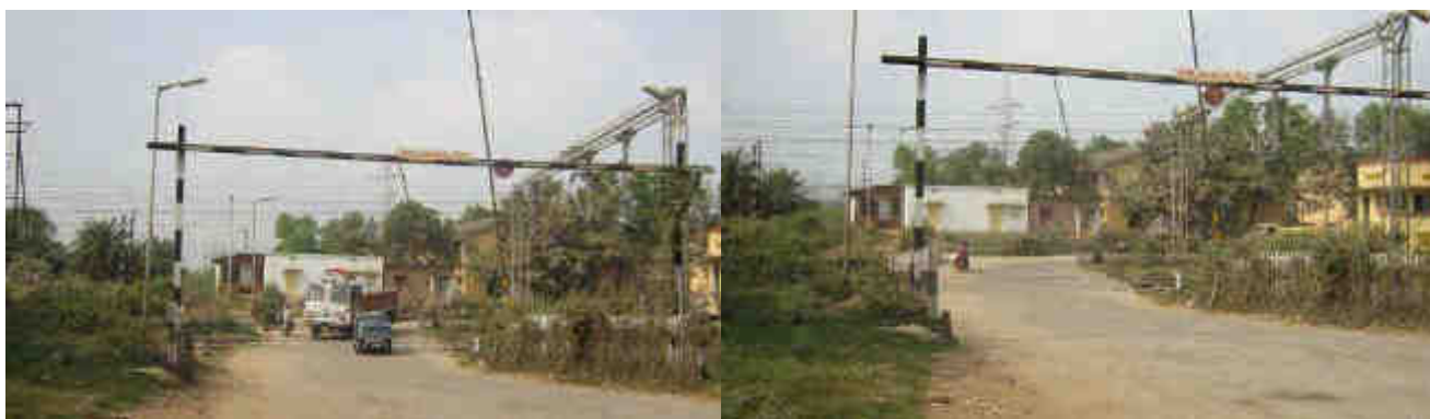
Accident prone area (Level Crossing)
