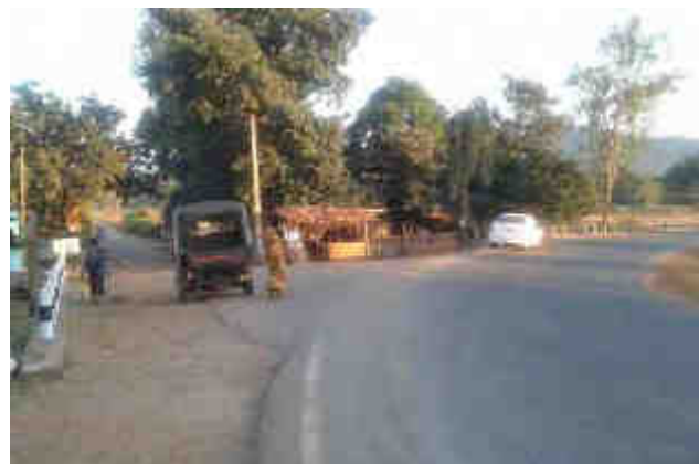
Side road joining on curve at Km 27+900
