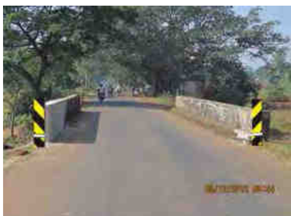
Culvert at Km 2+600
