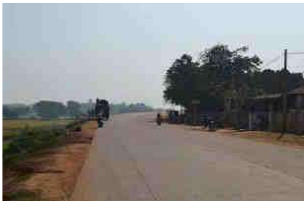
Approach to Major Bridge at high embankment
