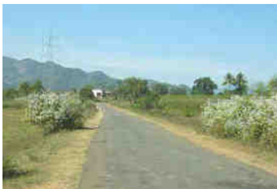
Road marking missing
