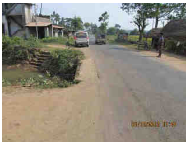
absence of parapet wall at Km 24+800
