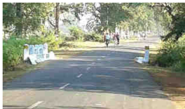
Parapets of Culvert/Bridge not delineated, Km 8+500 and Km 11+700
