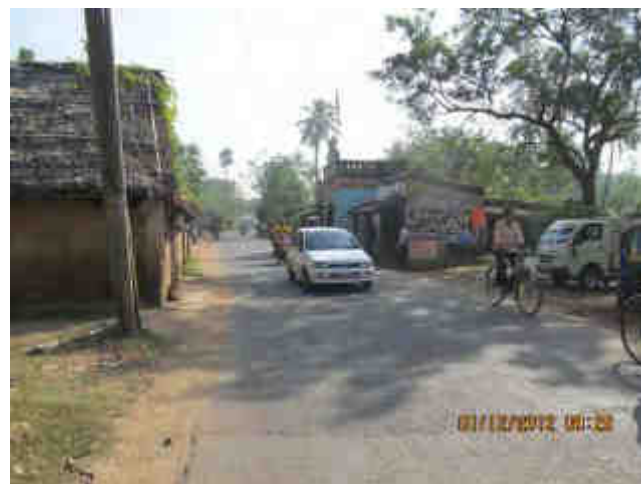
Built up area at Km 7+000
