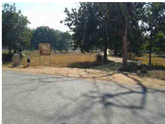
Side road joining with steep gradient Km 36+800
