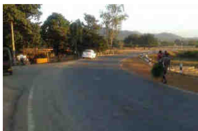
Sharp curve with BUA and access road (LHS), Km 27+900
