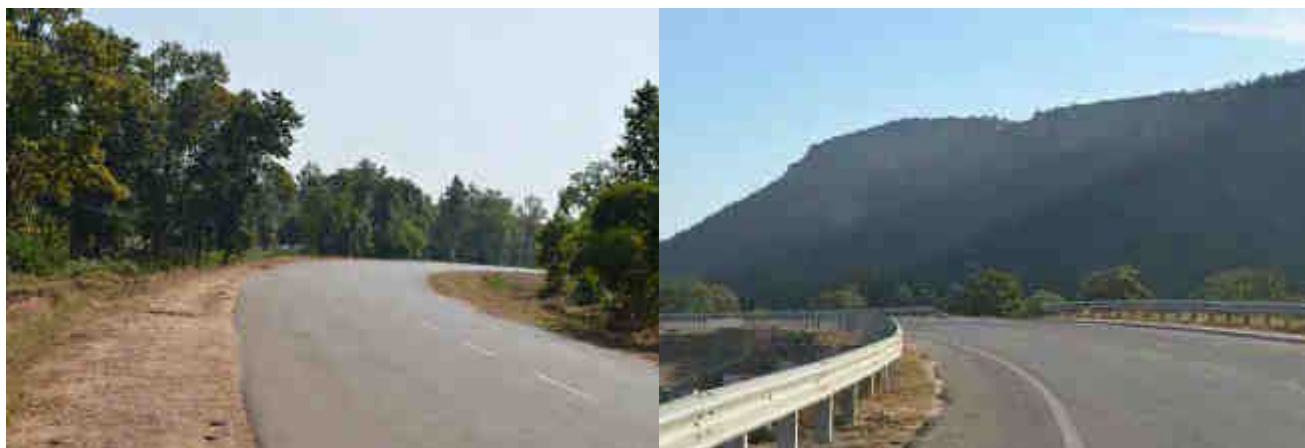
Curves on Project Road
