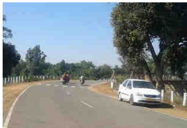
Bridge at Km 317+400, Sharp curve on approaches
