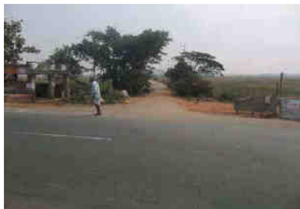
Absence of Centre line and edge line road marking at Km 225+480 and Km 219+500 respectively
