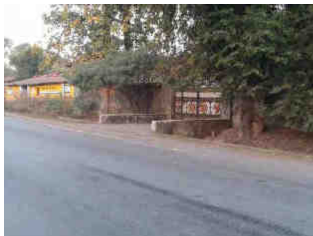
Deep drain and property access very near to the road edge, Km 74+000 to 75+000
