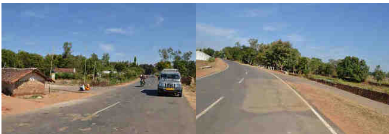
Skewed Side Road at Km 73+600 and Km 88+100
