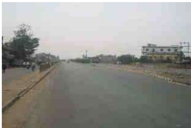
Absence of Centre line and edge line road marking at Km 225+480 and Km 219+500 respectively
