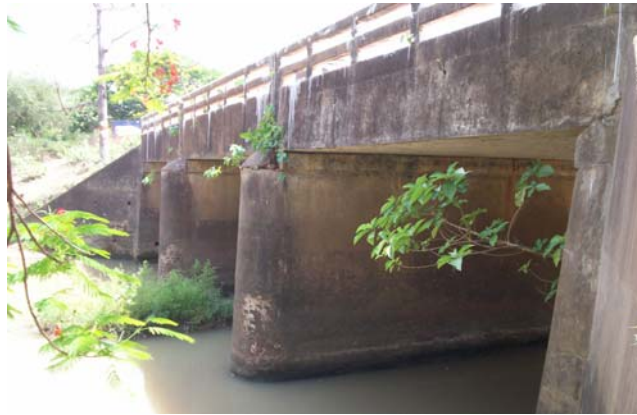
Bridge at Ch: 9/300
