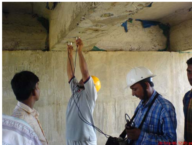
Pulse Velocity testing in RCC Girder for bridge at Ch.38/100
