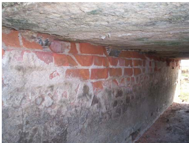
Bridge at Ch: 30/050
