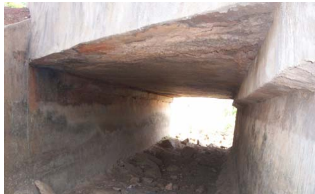
Bridge at Ch: 9/800
