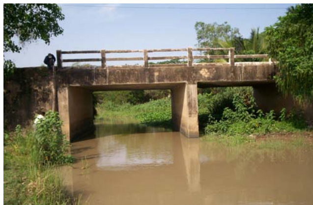
Bridge at Ch: 30/200
