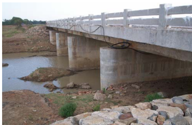
Bridge at Ch: 38/200
