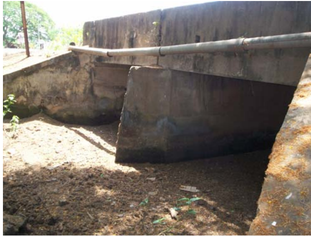
Bridge at Ch: 1/005
