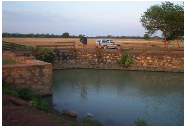
Bridge at Ch: 30/950
