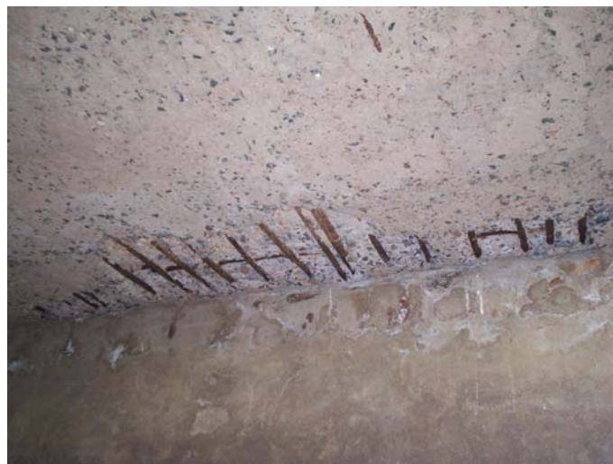
Bridge at Ch: 18/400
