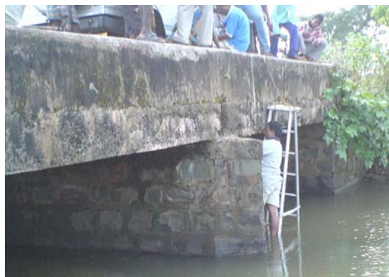
Pulse velocity testing in Deck slab for bridge at Ch. 38/200
