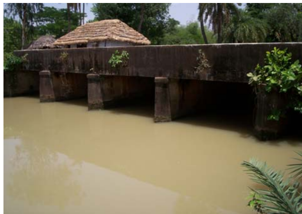
Bridge at Ch: 6/050
