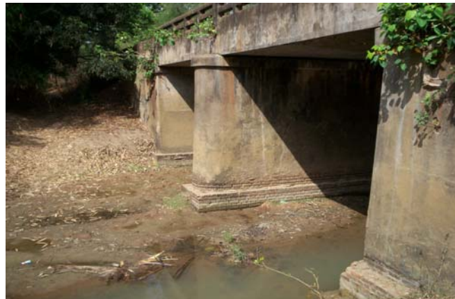
Bridge at Ch: 17/700
