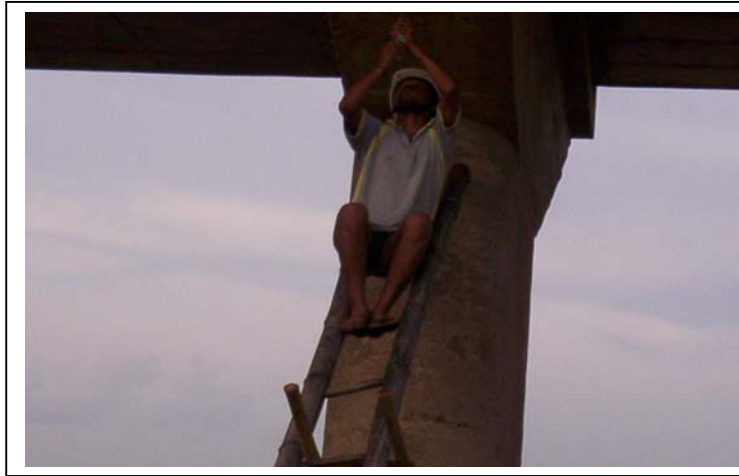
Rebound Hammer testing in Pier cap for bridge at Ch. 27/850
