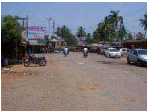
Poorly laid out major 4 arm junction
