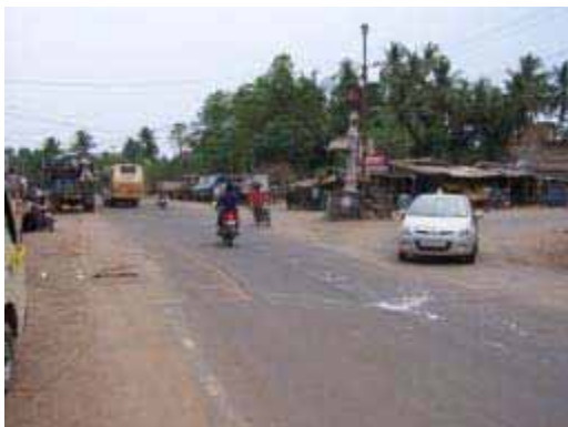
Hazardous 3 armed junction form
