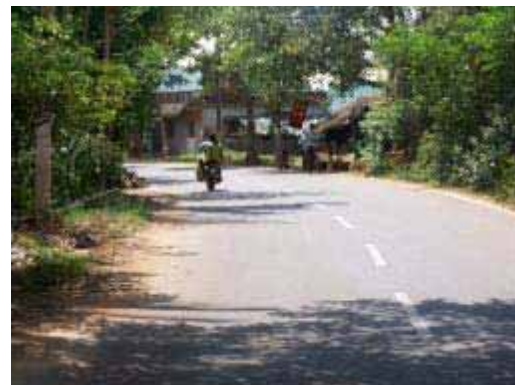
Sharp curve, but no warning signs
