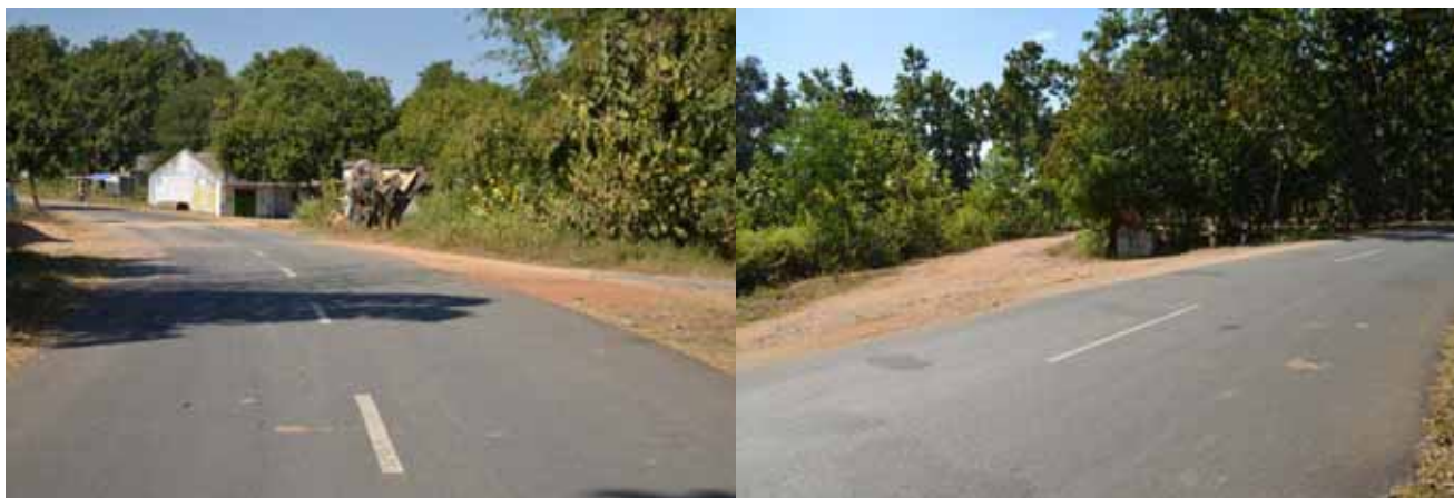
Skewed Side Road at Km 42+900 and Km 45+800
