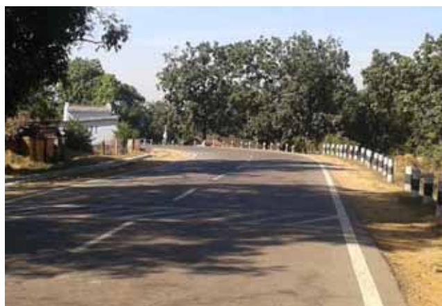
Sharp curve at Km 39+900
