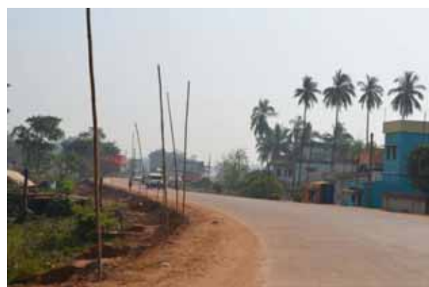
Curve at Km 8+600
