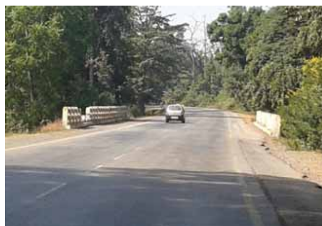
No edge protection on approaches of ROB at Km 49+900 and Bridge at Km 101+600
