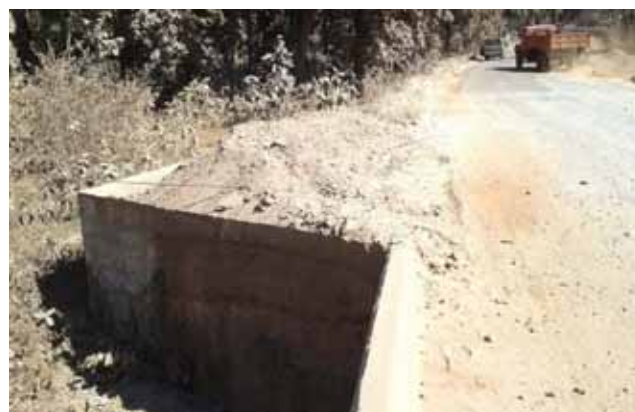
Unprotected approaches to the causeway, Km 24+000
