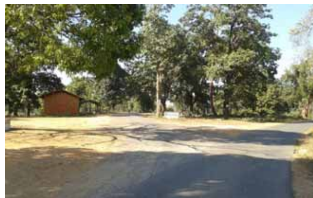
Side road joining on curve, Km 170+100
