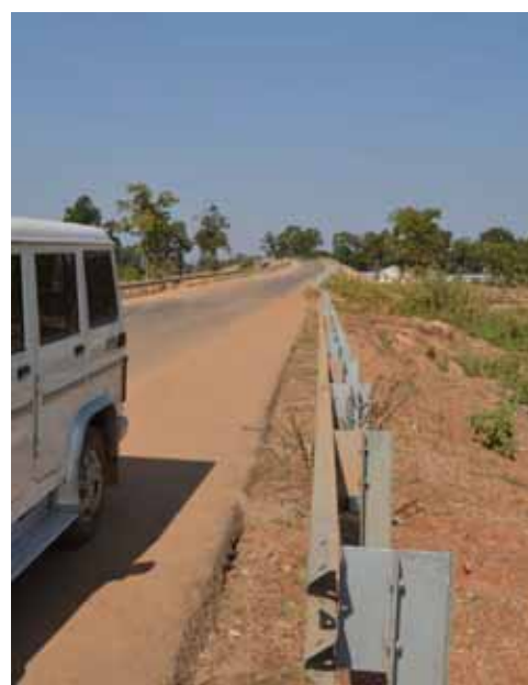
Crash Barrier very near to pavement edge
