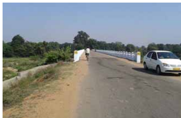
Bridge at Km 20+600, No protection on approaches
