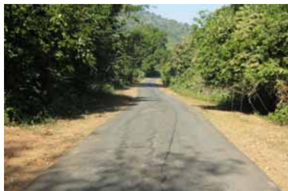
Road marking missing
