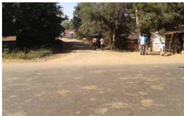
Restricted visibility from access road due to buildings and trees on corners, Km 312+900
