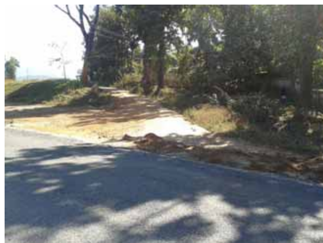
Side road joining at skew angle Km 24+350
