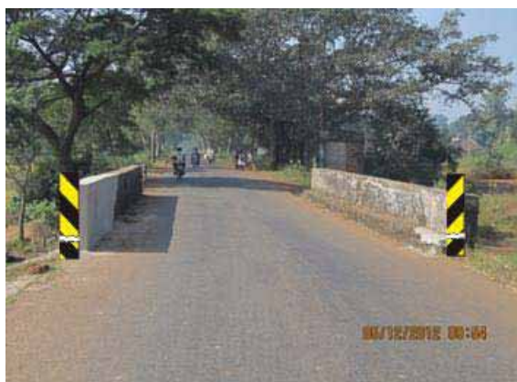
Culvert at Km 2+600
