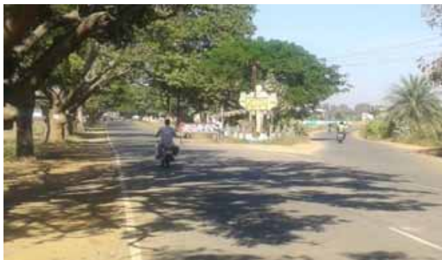
Km 316+900, intersection of NH-49 with Kuchinda town road (south of Kuchinda) – non-standard island with buildings and trees obstructing visibility
