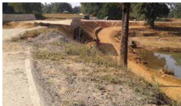
Sharp curve on high embankment without edge protection near approaching culvert (under construction), Km 31+800
