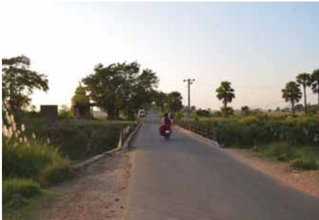
Missing bridge approach protection at Km 9+600
