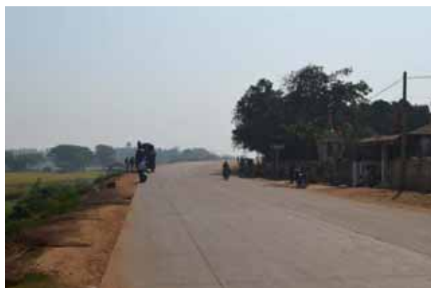
Approach to Major Bridge at high embankment
