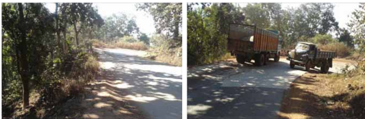
Km 19+250, dangerous hairpin bend
