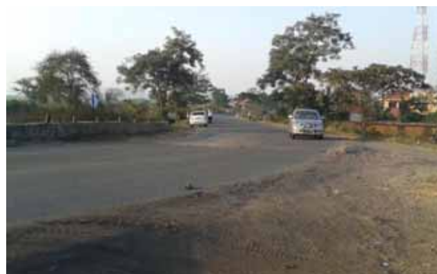
Traffic approaching sharp curve and ROB (view from the Access Road)
