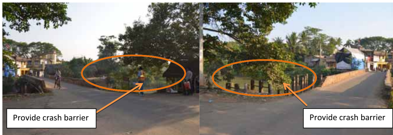
Junction at Km 4+950
