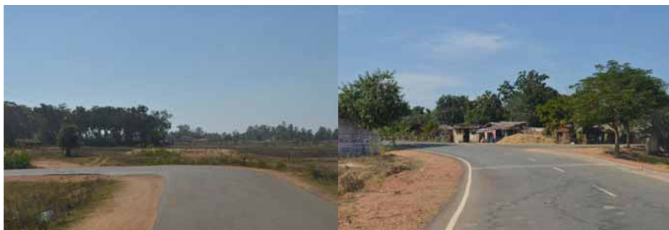
Sharp Curves on Project Road at Km 80+000 and Km 75+200
