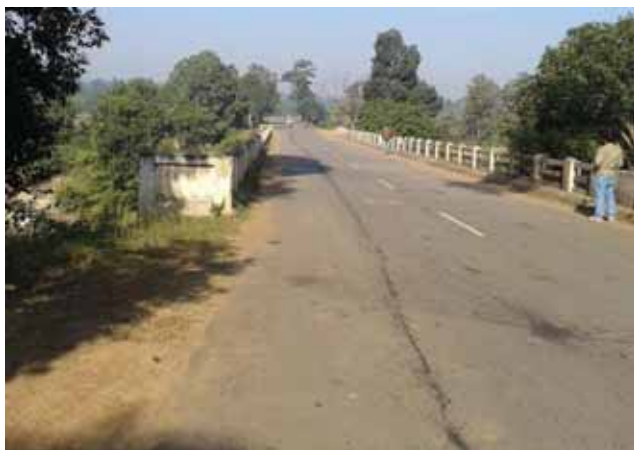
Parapets of culvert/bridge not delineated, Km 6+500 and Km 9+400
