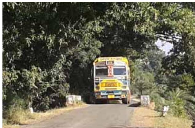
Parapets of Culvert/Bridge not delineated, Km 172+700 and Km 187+700
