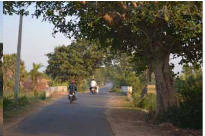
Culvert at Km 10+000
