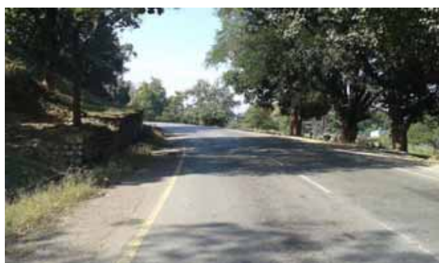
Sharp curve where visibility is obstructed due to wall and trees (on LHS), Km 107+800
