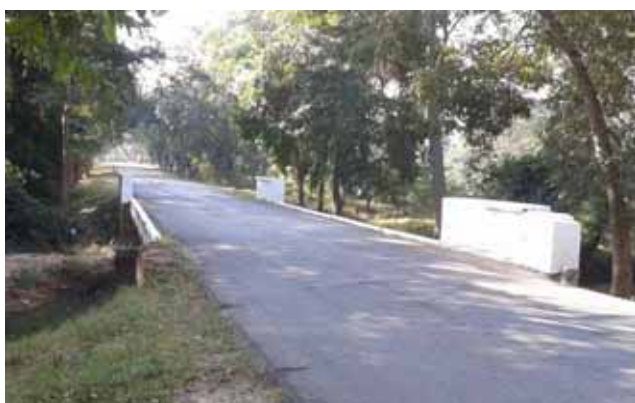
Parapets on Culvert/Bridge highly unsafe for VRUs as well as other traffic, Km 2+700 and Km 8+800
