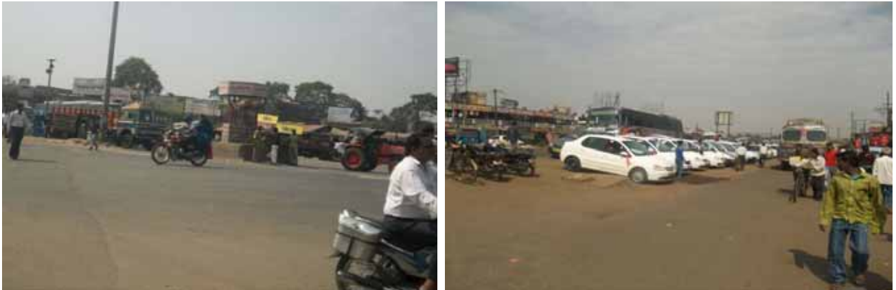
Poor junction layout and on street parking at roundabout at Km 219+000
