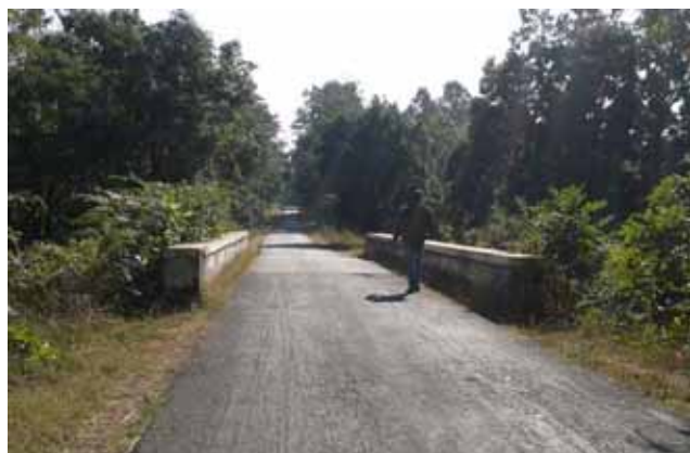
Parapets of Culvert/Bridge not delineated, Km 172+700 and Km 187+700
