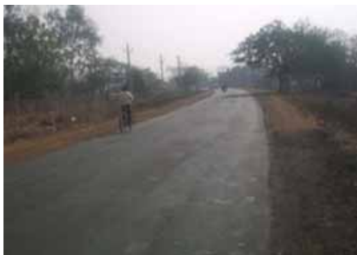
Curve at Km 6+500
