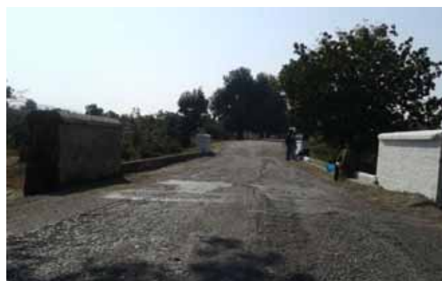
Parapets on Culvert/Bridge highly unsafe for VRUs as well as other traffic, Km 2+700 and Km 8+800
