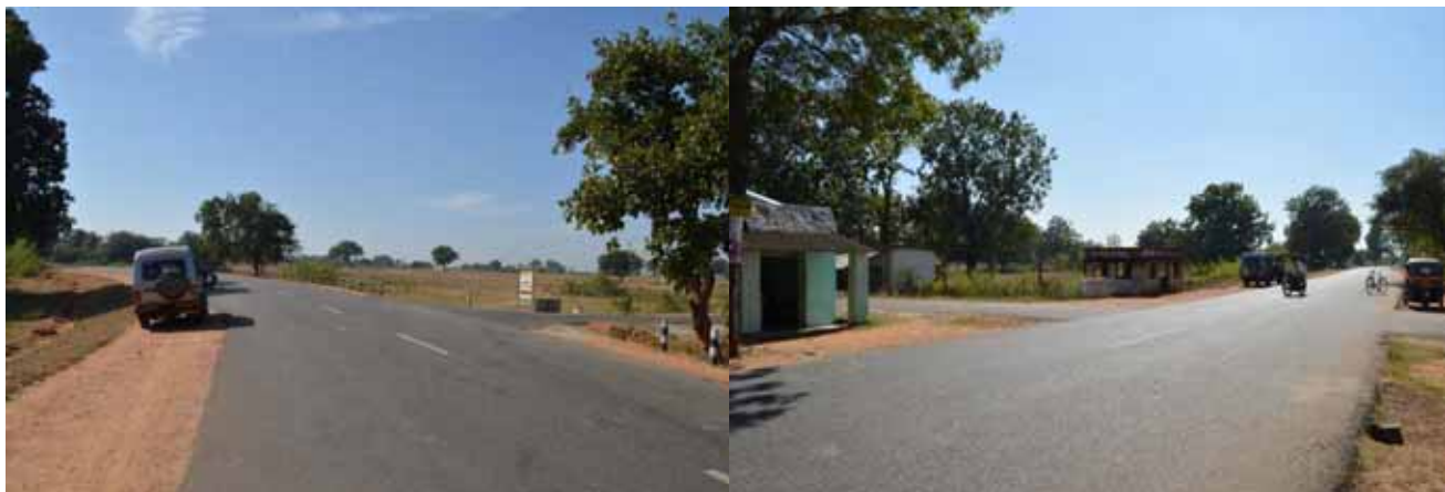
Minor Junctions at Km 66+950 and at Km 76+800
