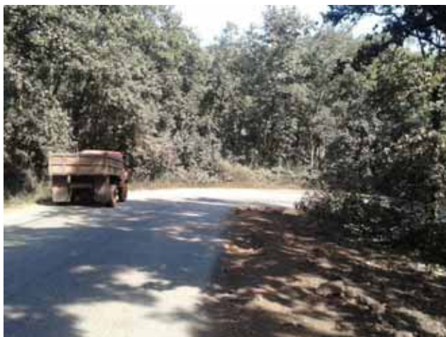
Hairpin bend with steep gradient at Km 22+100
