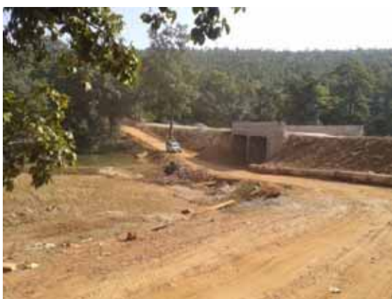
Km 31+800 – Traffic diversion at the site of construction of culvert
