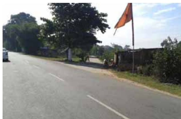
Side road joining at acute angle, Km 4+600
