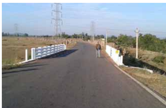
Parapets of Culvert/Bridge not delineated, Km 38+500 and Km 30+200
