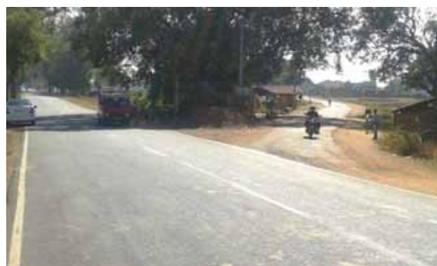
Access road joining NH-49 at skew angle, Km 319+800
