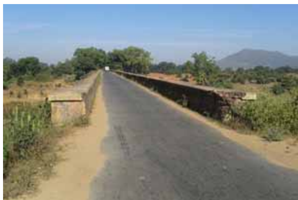
Parapets of bridge not delineated, Km 313+300 and Km 317+400
