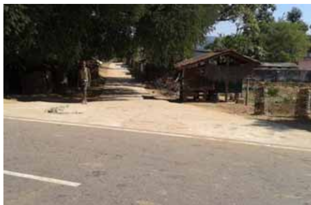
Side road joining with steep gradient at Km 27+000
