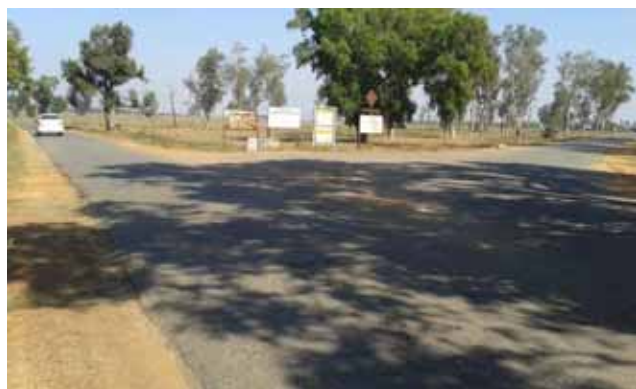
Side road joining at skew angle Km 157+400
