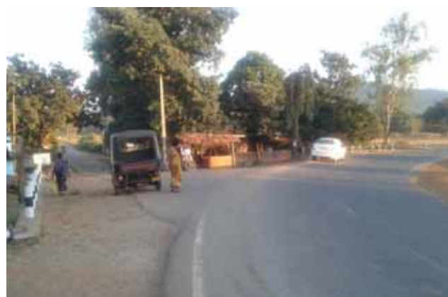
Side road joining on curve at Km 27+900
