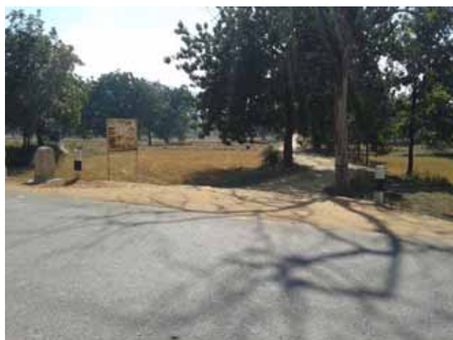
Side road joining with steep gradient Km 36+800
