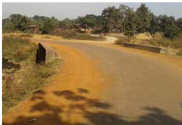
Parapets of Culvert/Bridge not delineated, Km 6+200 and Km 0+600
