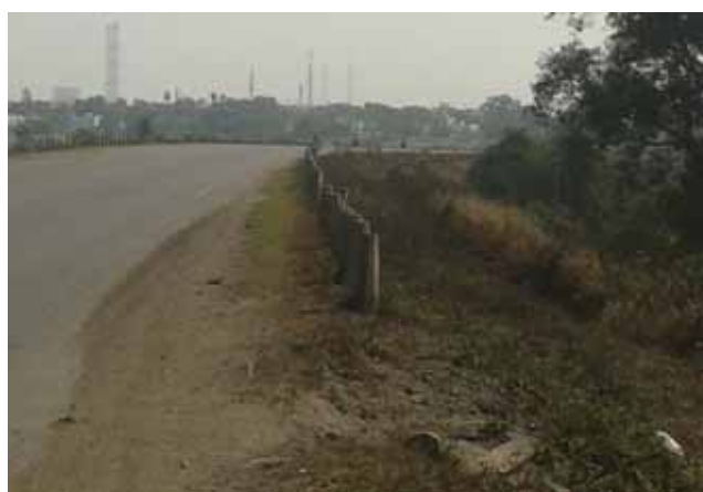
No edge protection on approaches of ROB at Km 49+900 and Bridge at Km 101+600
