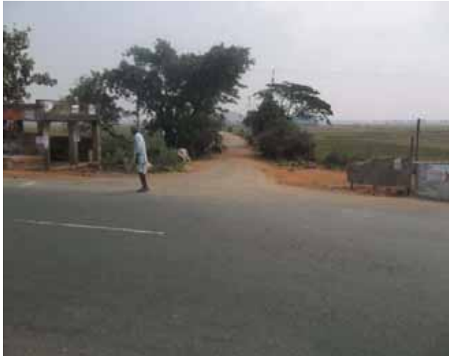
Side road with poor visibility due to vegetation at Km 225+200
