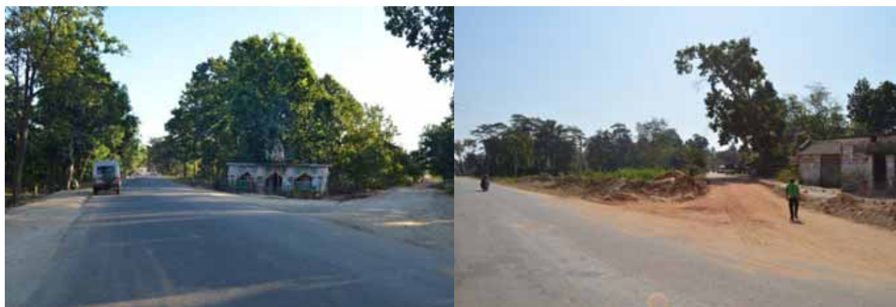
Skewed Side Road at Km (Section I) and Km 10+500 (Section II)
