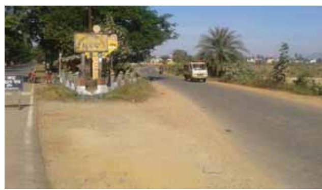
Km 316+900, intersection of NH-49 with Kuchinda town road (south of Kuchinda) – non-standard island with buildings and trees obstructing visibility
