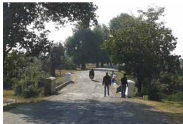
Parapets of Culvert/Bridge not delineated, Km 13+700 and Km 8+800
