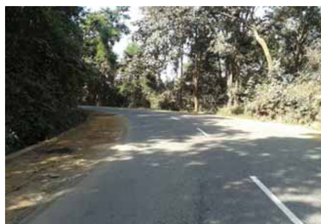
Sharp curve in ghat section at Km 30+200
