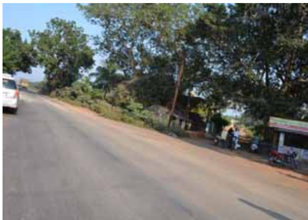
Skewed Side Road at Km 5+800
