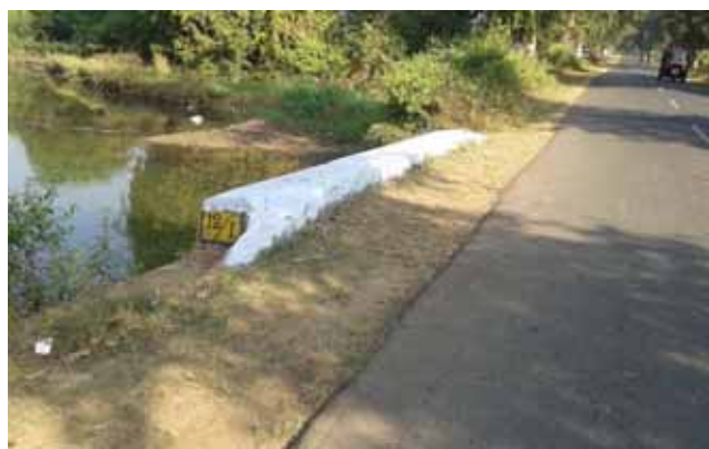
No parapets on Culvert/Bridge highly unsafe for VRUs as well as other traffic, Km 12+000 and Km 20+000
