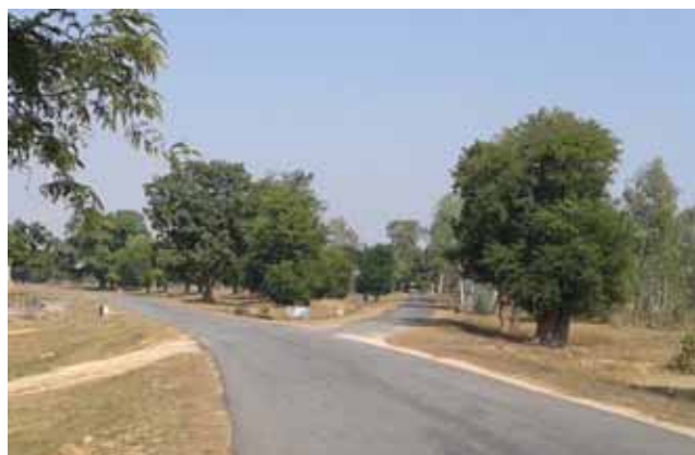
Side road joining at skew angle Km 21+000
