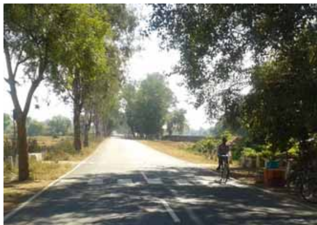
Trees very near the road edge, Km 319-320
