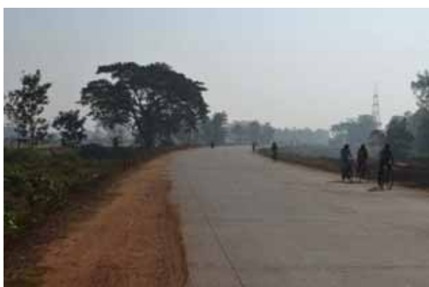
Curve at Km 4+400
