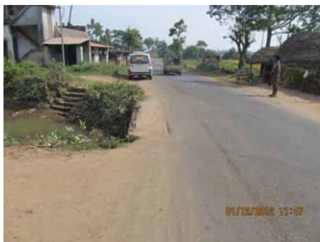
absence of parapet wall at Km 24+800
