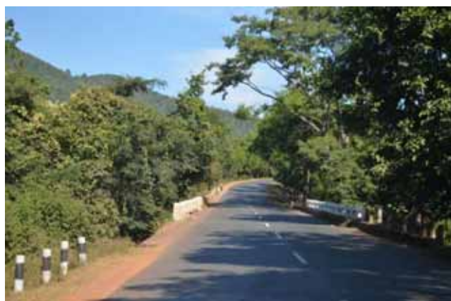
Absence of OHM and absence of approach protection at Km 461+800 and Km 470+250
