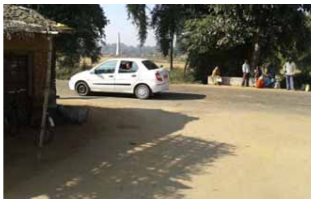
Side road joining at Km 7+100 – visibility restricted due to buildings on both the corners(view from side road)
