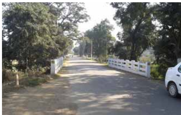
Parapets of Culvert/Bridge not delineated, Km 3+300 and Km 9+300
