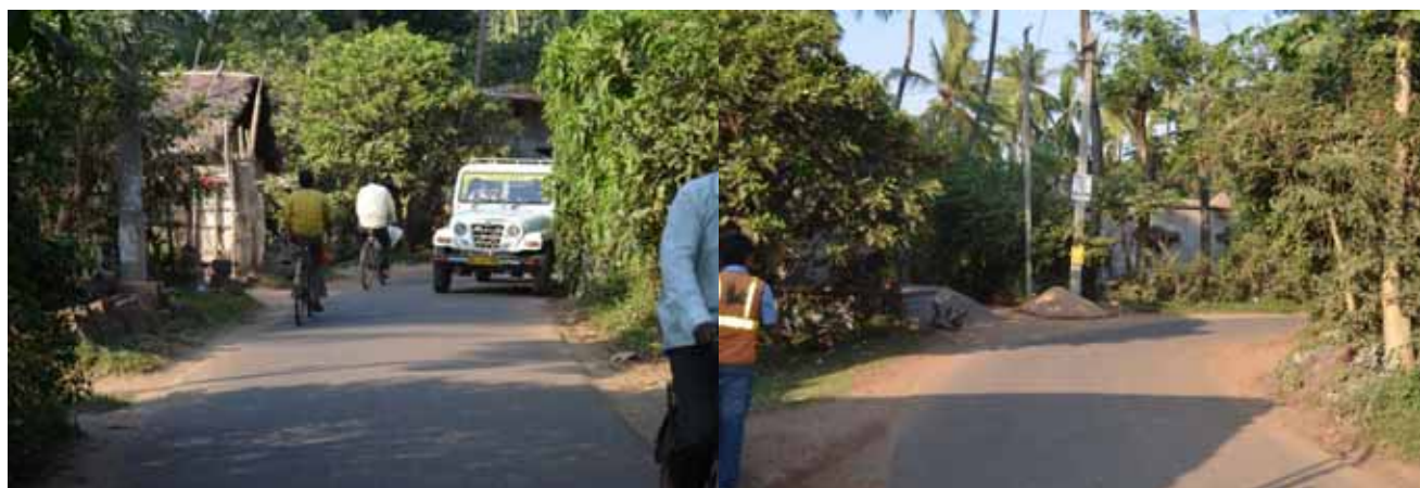
Sharp Curves on Project Road at 1+300 and 1+450
