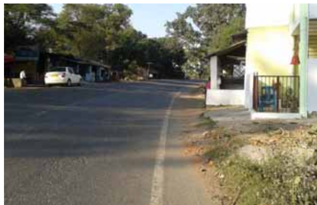
Buildings very close to edge of road in BUA, Km 62-63 Talpatia village
