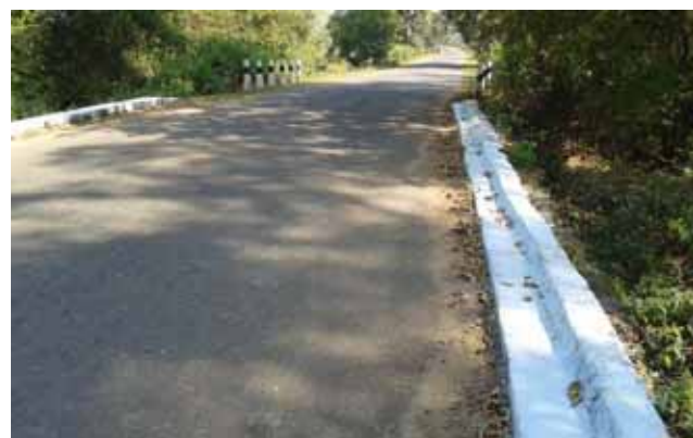
No parapets on Culvert/Bridge highly unsafe for VRUs as well as other traffic, Km 12+000 and Km 20+000
