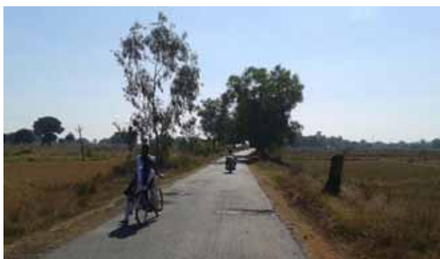
Photographs of SH-24 in rural and urban areas where no road markings are provided (Km 154 to 155, and Km 155 to 156)
