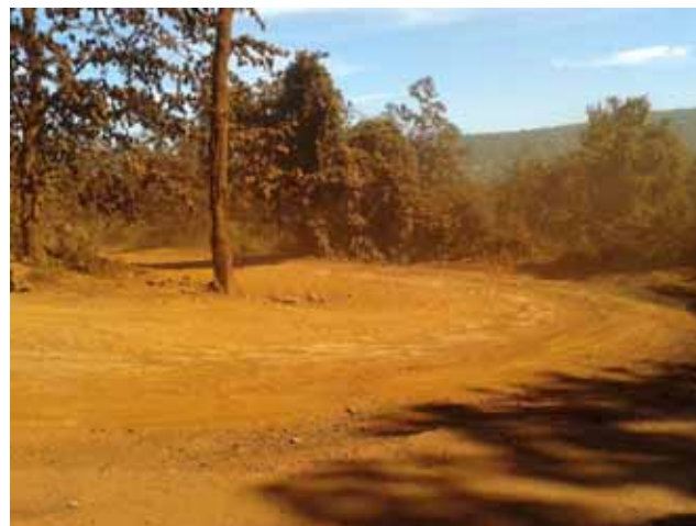
Hairpin bend with poor road condition at Km 11+400
