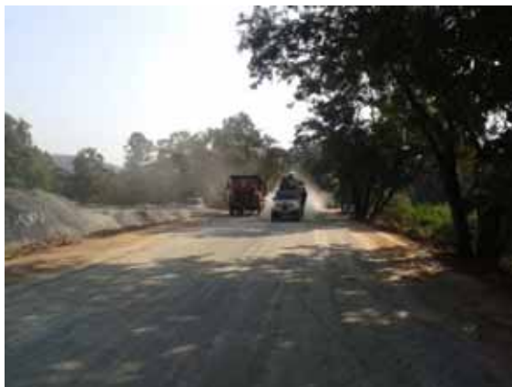
Road construction Km 35+000 to 36+000
