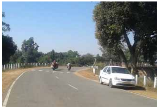
Bridge at Km 317+400, Sharp curve on approaches
