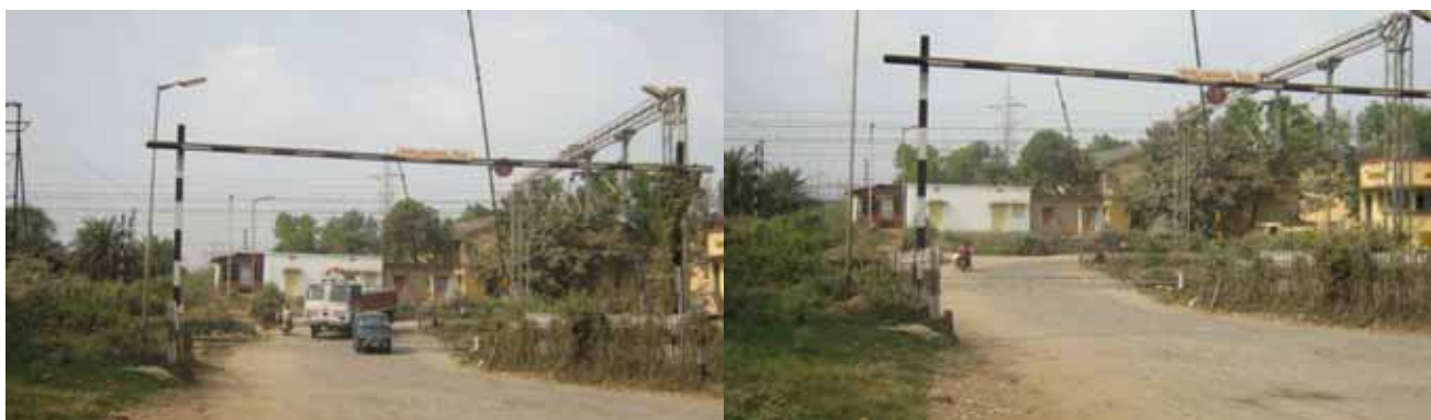
Accident prone area (Level Crossing)
