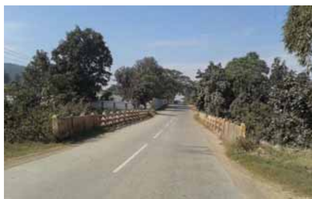
Parapets of Culvert/Bridge not delineated, Km 3+300 and Km 9+300
