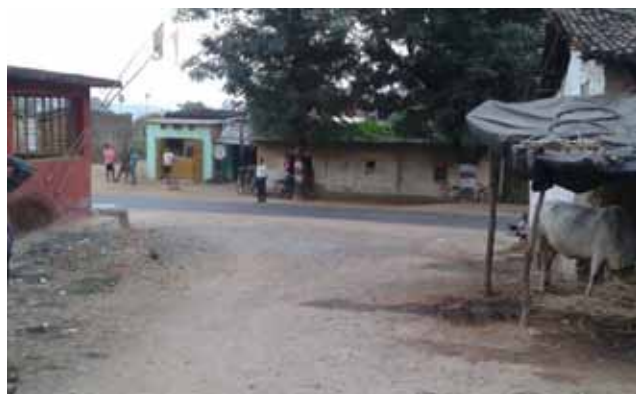
Restricted visibility from access road due to buildings on corners, Km 6+500
