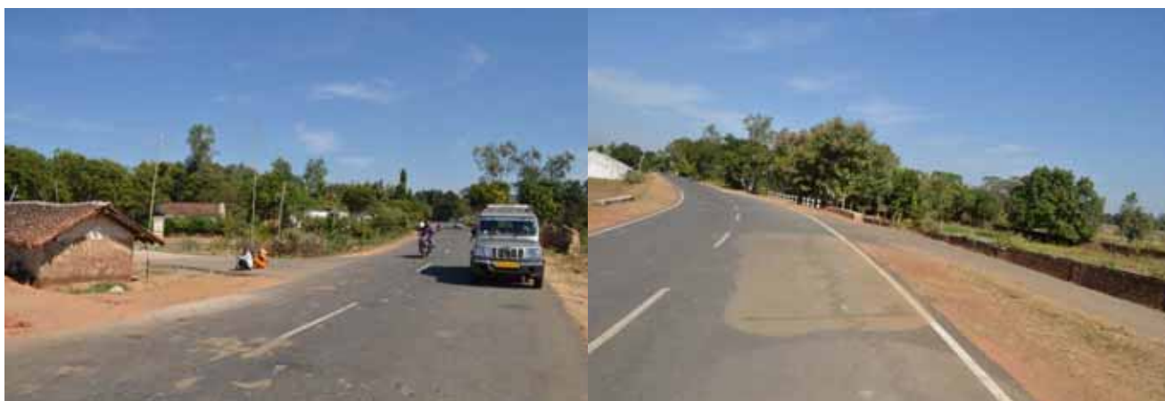
Skewed Side Road at Km 73+600 and Km 88+100
