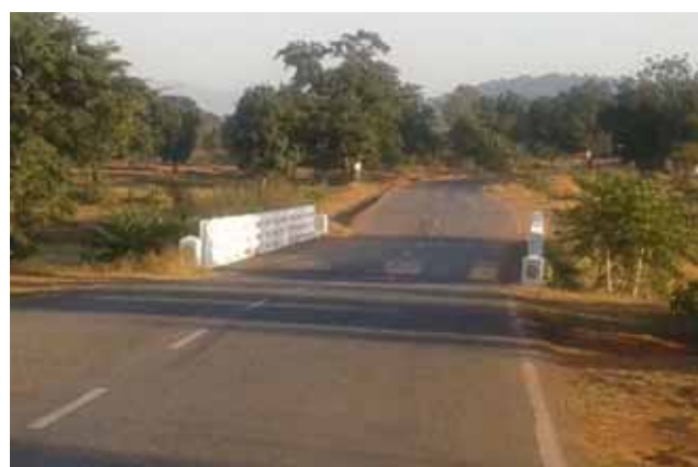
Parapets of Culvert/Bridge not delineated, Km 38+500 and Km 30+200
