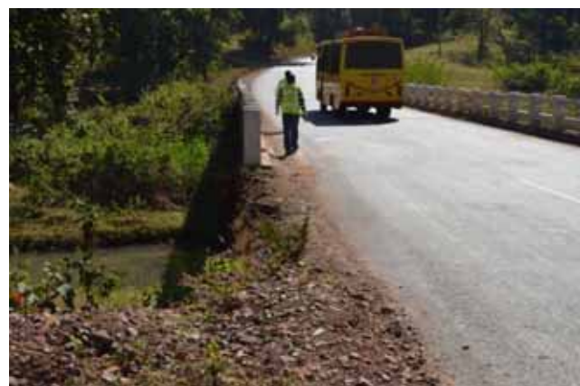
Absence of OHM and absence of approach protection at Km 461+800 and Km 470+250
