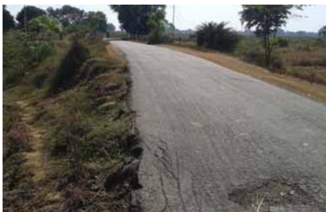
Poor condition of earthen shoulder, Km 155-156 and Km 191-192
