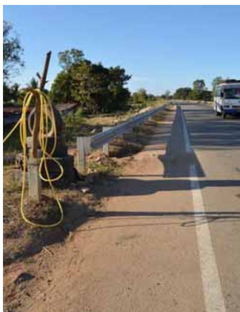
Crash Barrier very near to pavement edge
