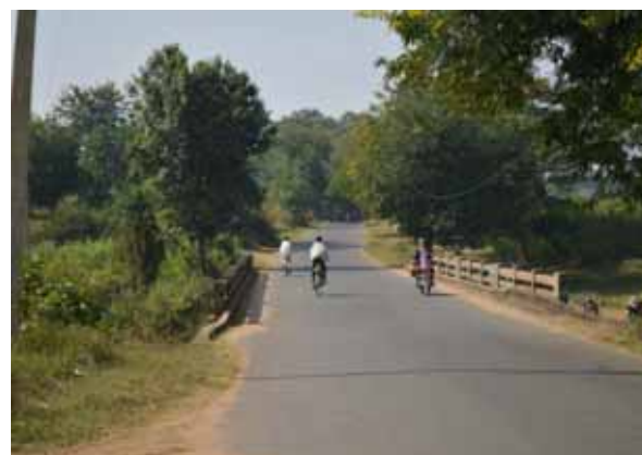
Minor Bridge at Km 48+700
