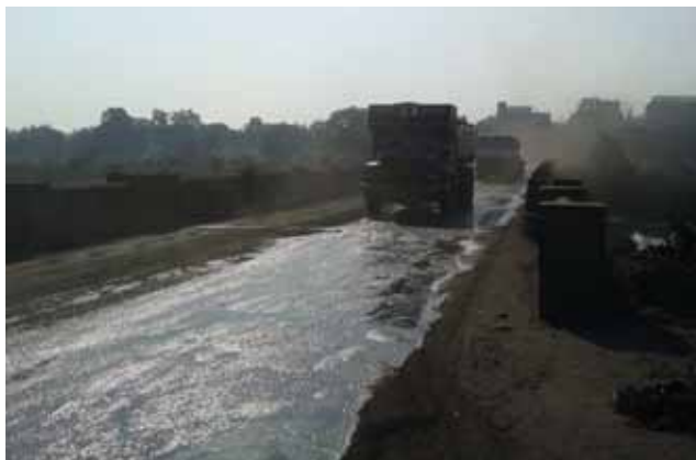
Parapets of Bridge not delineated, Km 32+200 and Km 165+400
