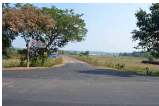
Side roads perpendicular to Major Road at Km 16+900
