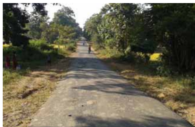
Poor condition of earthen shoulder, Km 155-156 and Km 191-192
