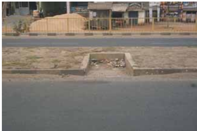
Drain located near to pavement edge at Km 219+100
