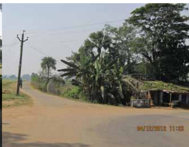
Side roads skewed to Major Road at Km 22+650
