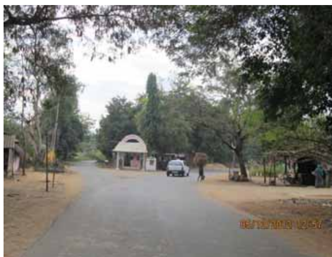
Skewed Side road at Km 28+850
