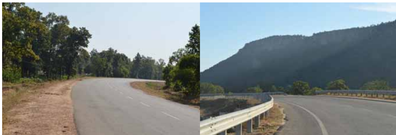
Curves on Project Road
