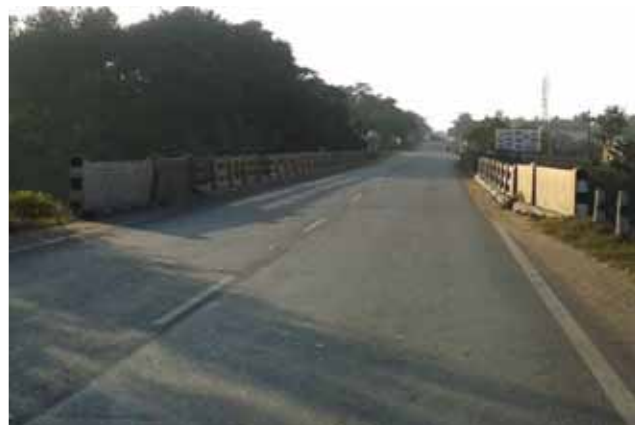
Parapets of Bridge not delineated, Km 32+200 and Km 165+400
