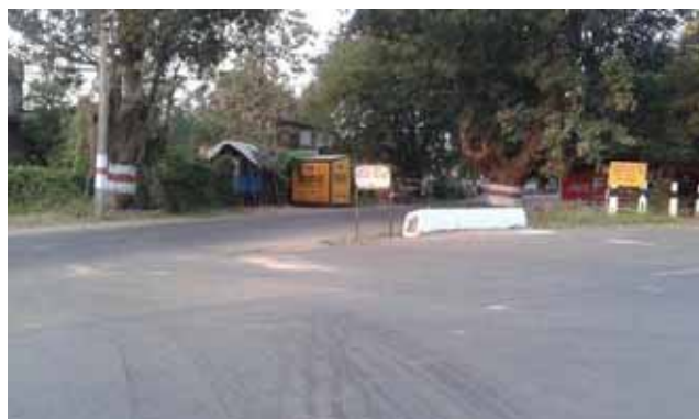
Km 5+100 intersection of SH-15 with link road - lack of road markings and delineation
