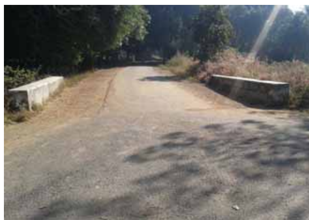
Parapets of culvert/bridge not delineated, Km 6+500 and Km 9+400
