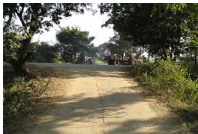
Side Road joining SH-10 at steep gradient, Km 12+900
