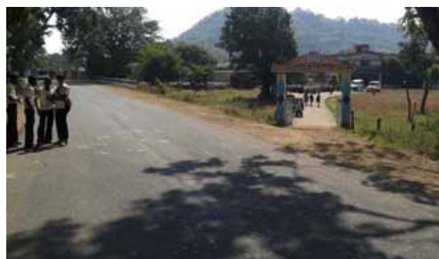
Access road joining SH-15 at skew angle and with steep gradient, Km 24+200
