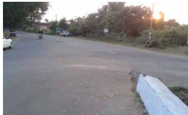
Km 5+100 intersection of SH-15 with link road - lack of road markings and delineation
