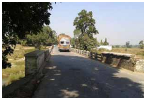
Parapets of Culvert/Bridge not delineated, Km 13+700 and Km 8+800
