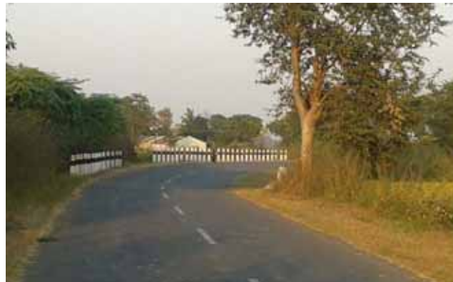
Image 1.1: Sharp curve with restricted visibility at Km 0+400 and Km 3+800
