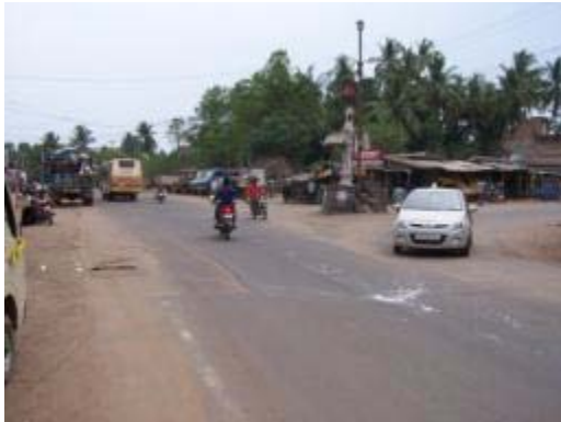
Hazardous 3 armed junction form
