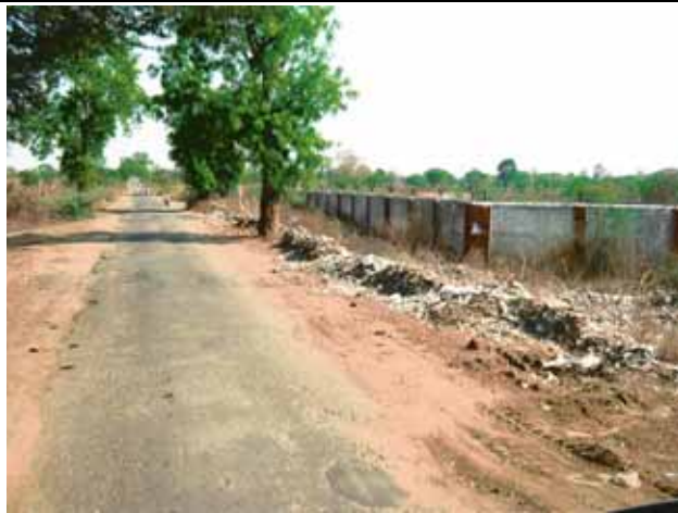
A9: Unclean road side
