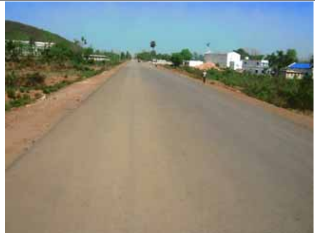
C8: Wide road with good surface
