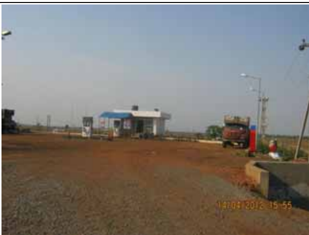
B29: Filling station on road side
