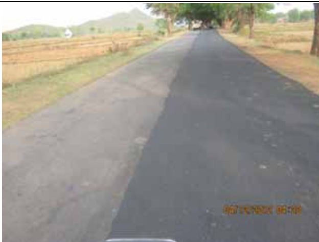
E23: Newly construction road surface
