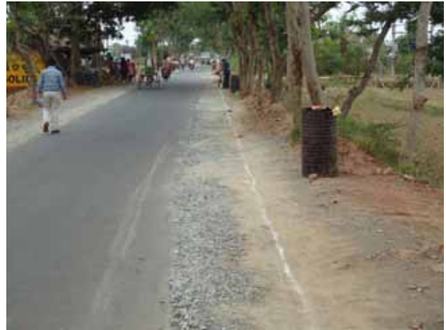
D8: Construction work in progress
