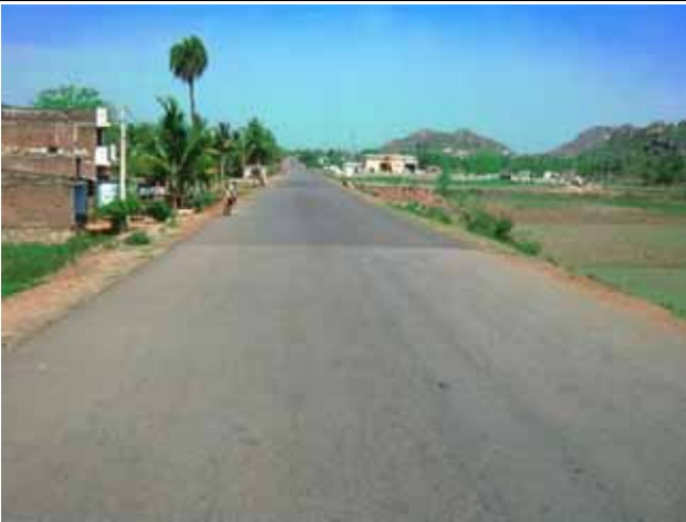
C3: Double lane road with good surface
