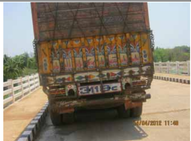
B6: Wrong Parking on the bridge
