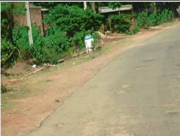
C9: Milestone on road side
