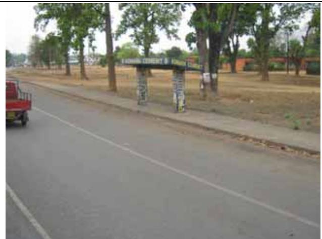
F24: Proper marking on the road
