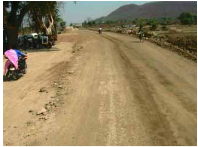
A20: Road construction in progress
