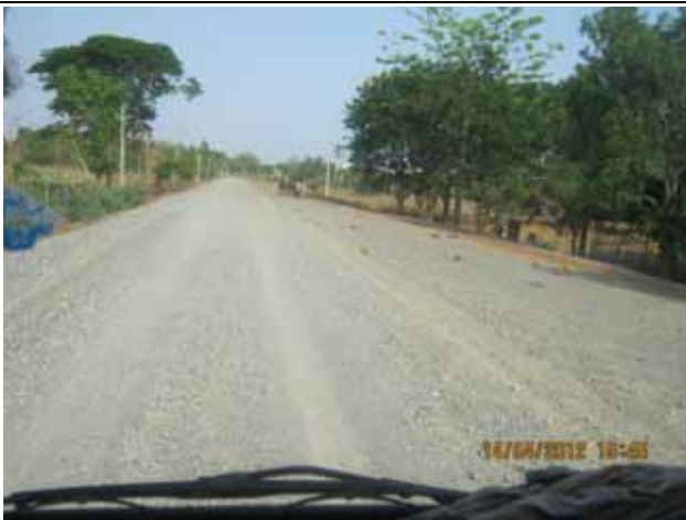
B27: Road widened and surfacing work done partially
