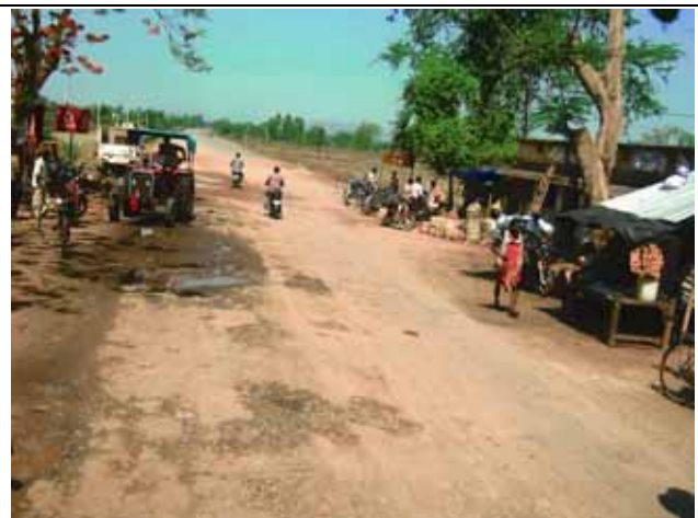
C12: Congested road with water logging
