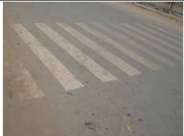
F16: Zebra crossing on the road
