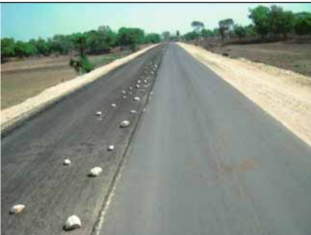
A23: Construction in progress
