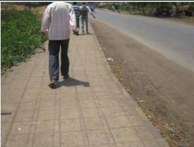
F15: Pedestrian-lane on road side
