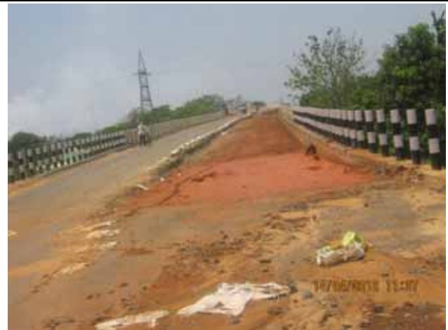
B4: Maintenance work on the bridge
