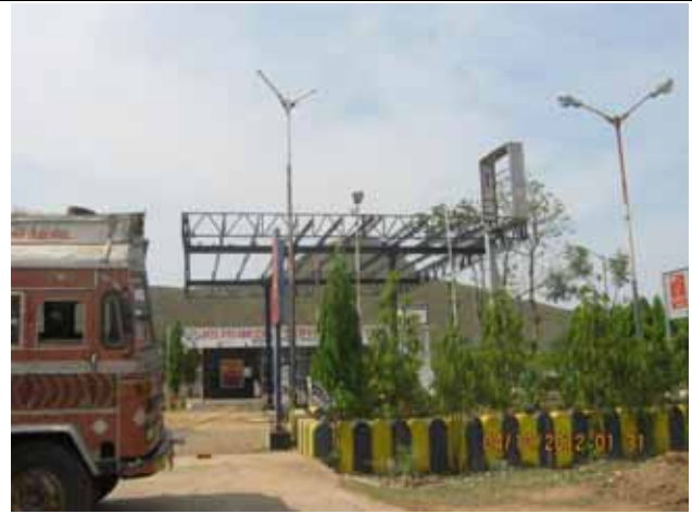
E14: Filling station on road side
