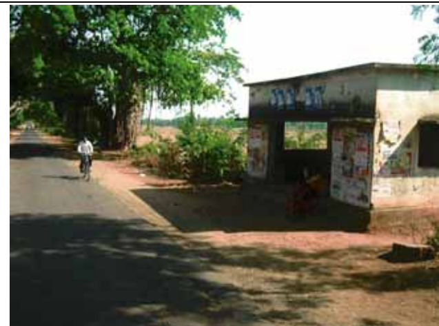
A12: Rain shelter-cum-bus stop on road side
