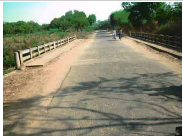
A6: Bridge on the road
