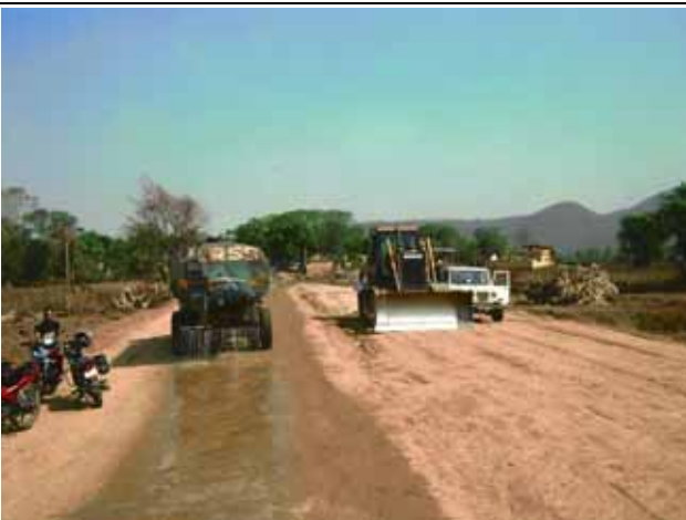
A17: Road construction work in progress
