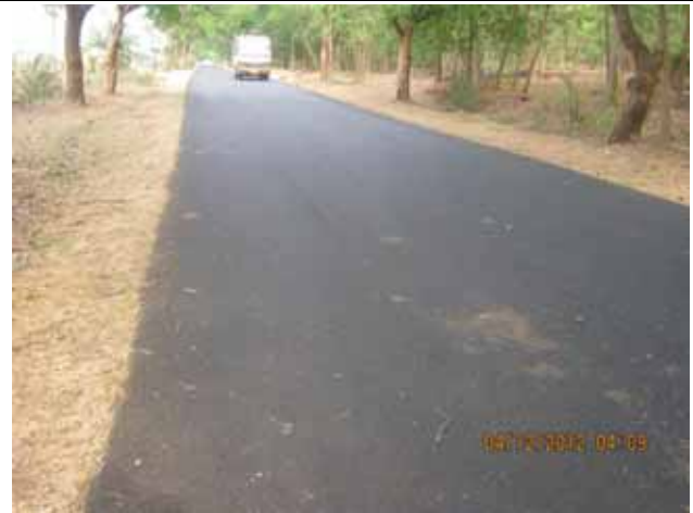
E22: Double lane road with good surface
