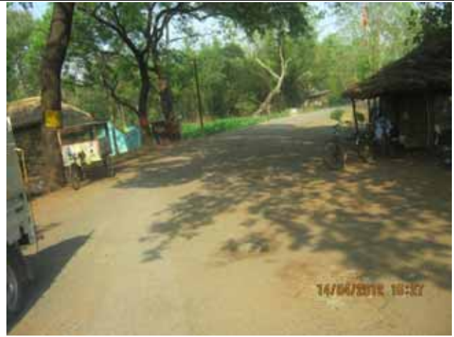
B20: Road encroachment
