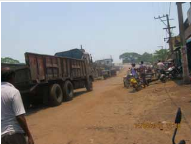
B5: Bad surface of the road
