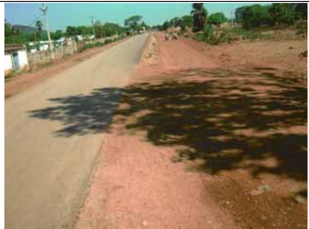
C6: Work in progress for double lane road
