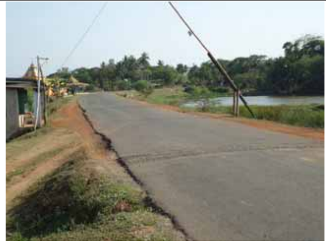
D14: Speed breakers on the road
