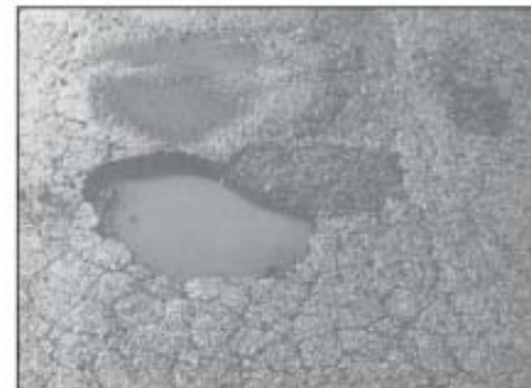
High Severity Pothole
