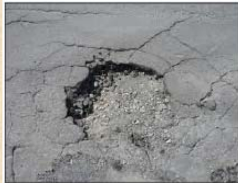
Medium Severity Pothole
