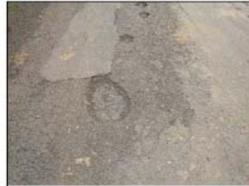
Low Severity Pothole
