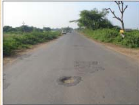
Low Severity Pothole
