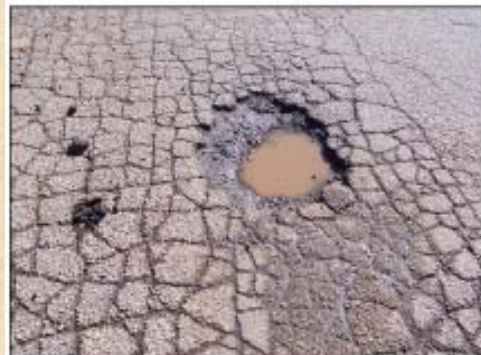
High Severity Pothole
