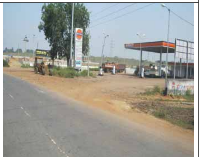
F18: Filling stations on road side
