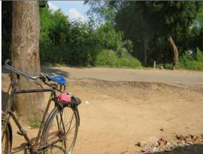
A7: Damaged edges of the road
