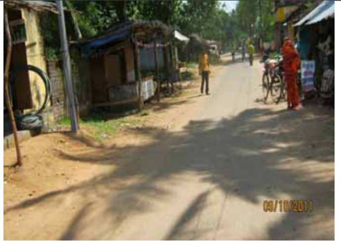
E2: Single lane road and road encroachment
