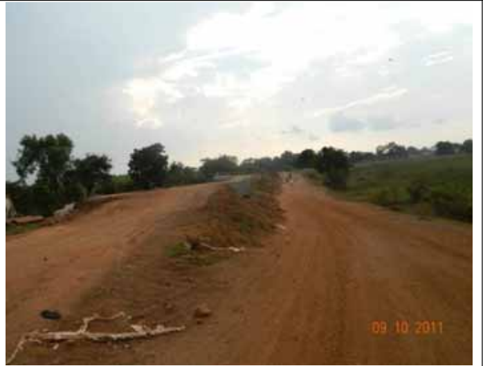
B8: Culvert/bridge work is under process
