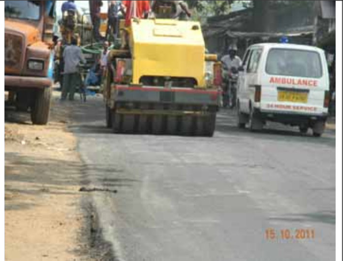
D2: Road work is going on this road
