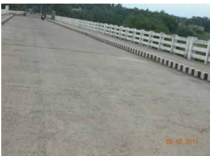
B17: Pavement on the flyover 2-3 km before Bhadrak
