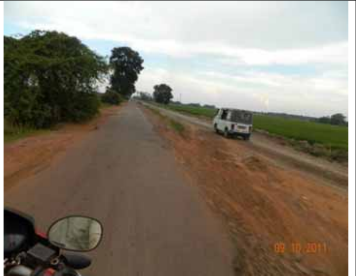
B14: Road widened and surfacing work done partially
