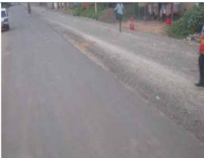
A23: Road widened and one lane completed
