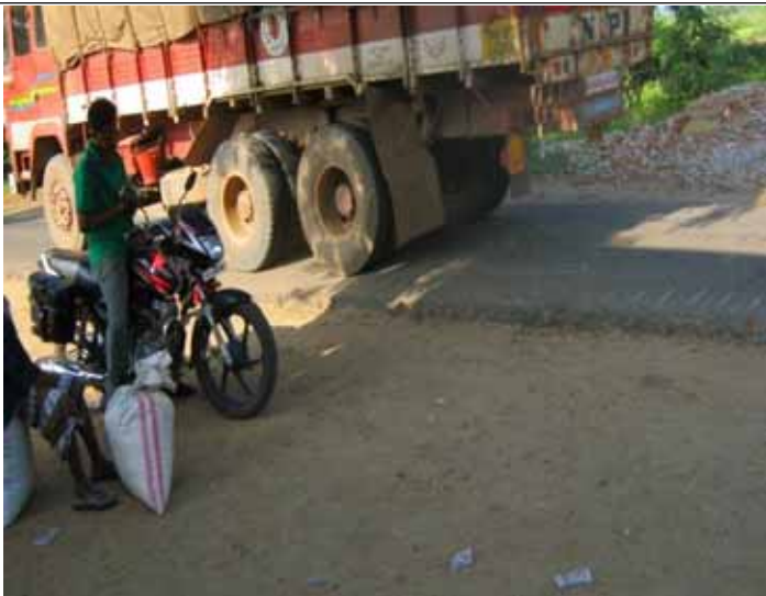
A15: Single lane road; difficult for the 2 nd vehicle to pass
