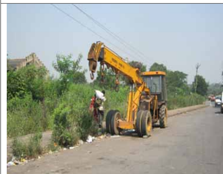
F11: Crane facility on the road
