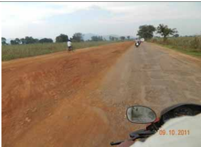
B5: Road widened but needs surfacing on this stretch
