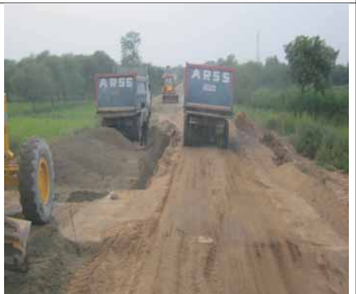
A22: Road construction process going on
