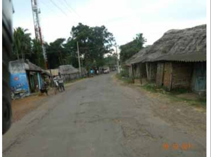
B18: Road encroachment
