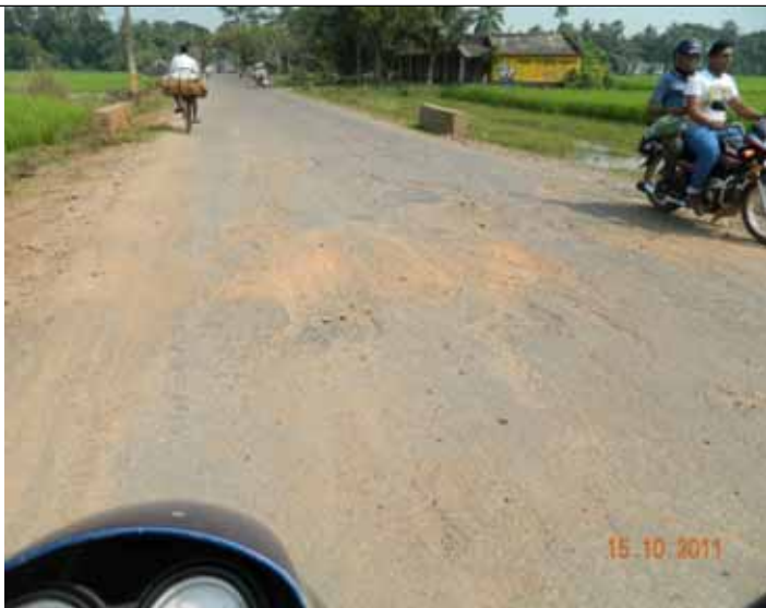
D9: Double lane road with surface is in bad condition
