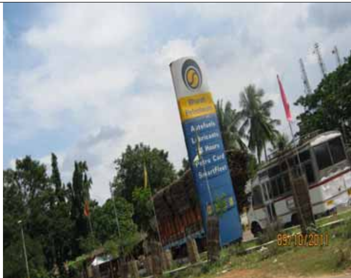
E11: Filling station on road side
