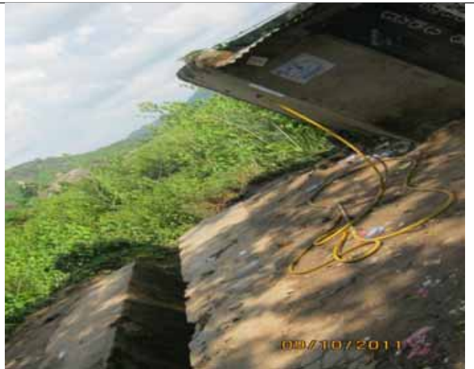
E4: Vehicle washing facility on the road side
