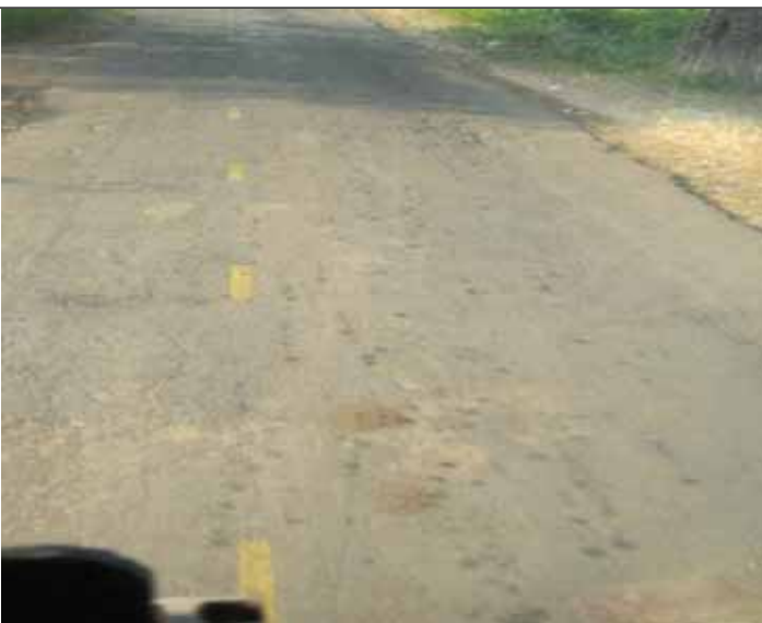
A17: Less visible road markings
