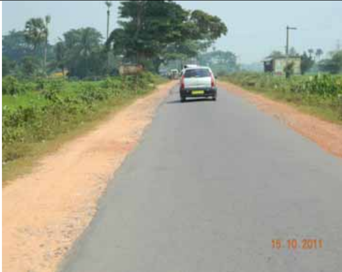
D7: Single lane, good surface road but edges are dangerous
