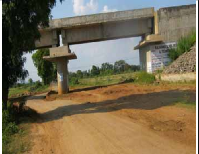
A8: Flyover on the road
