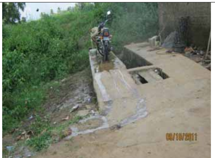
E6: Vehicle washing facility on the road side
