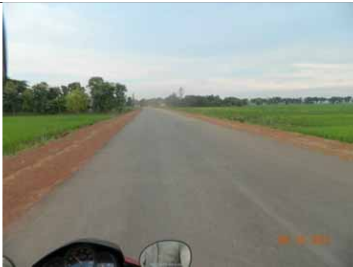
B9: Double lane complete with good surface
