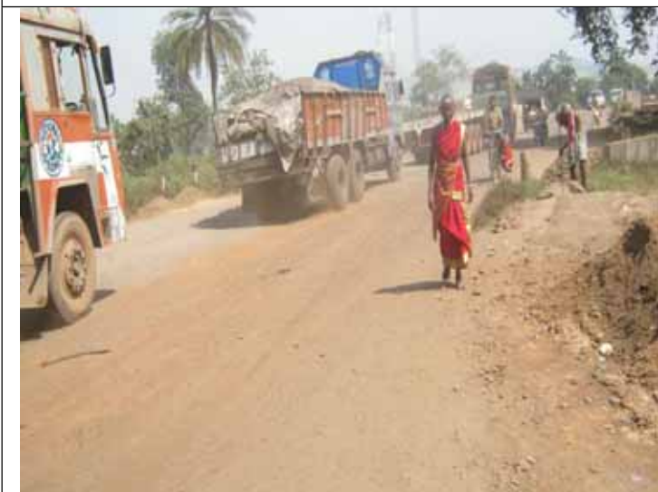
F9: Bad surface of the road
