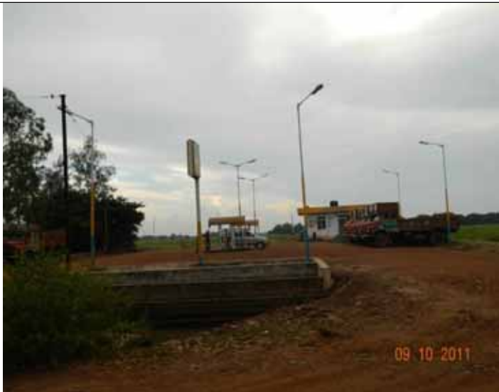
B15: Filling station on road side
