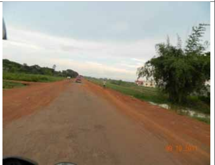
B10: Road widened but needs surfacing on this stretch
