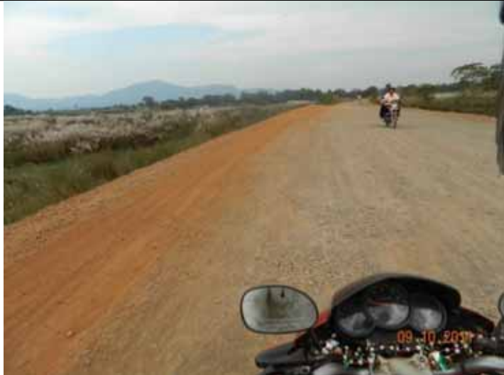
B7: Road widened and surfacing work done partially
