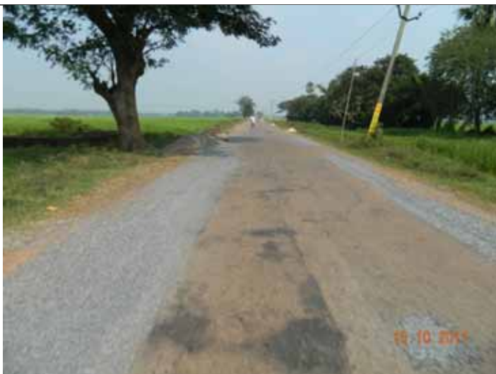
D11: Road maintenance work in progress
