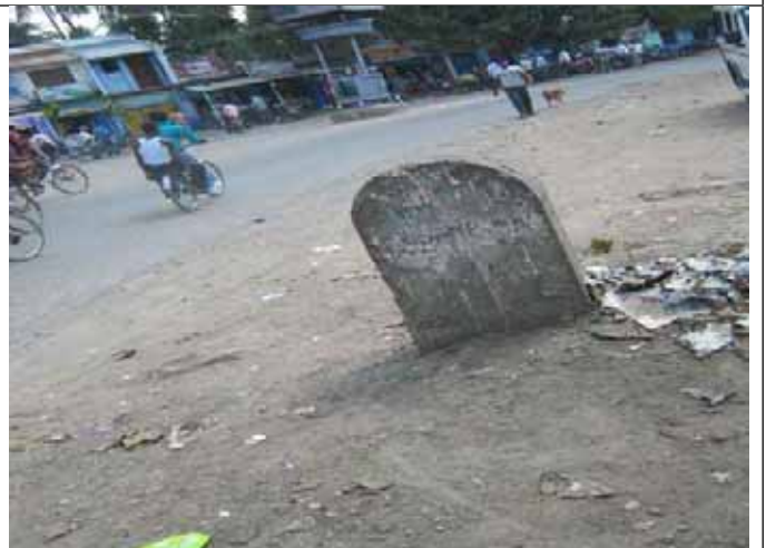
C18: Milestone on the road side with no information on it
