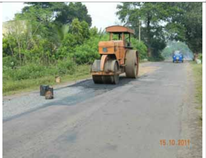
D12: Road maintenance work in progress
