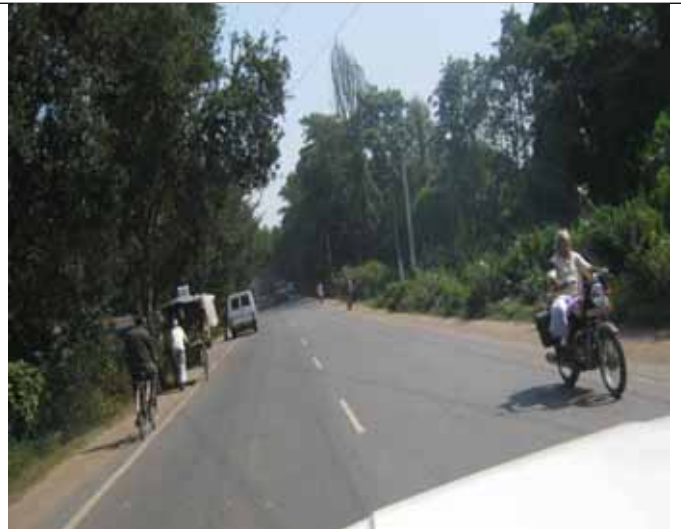
F4: Road markings on the road
