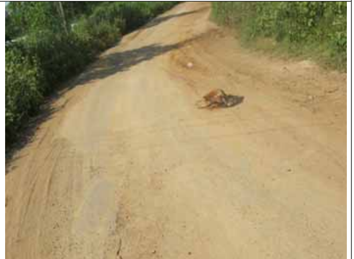
A4: No accident clearance on the road
