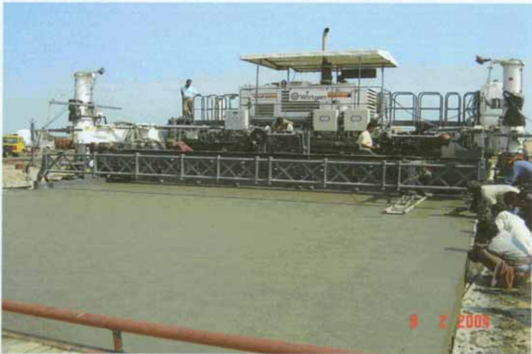
Laying, Compaction & finishing of Concrete
