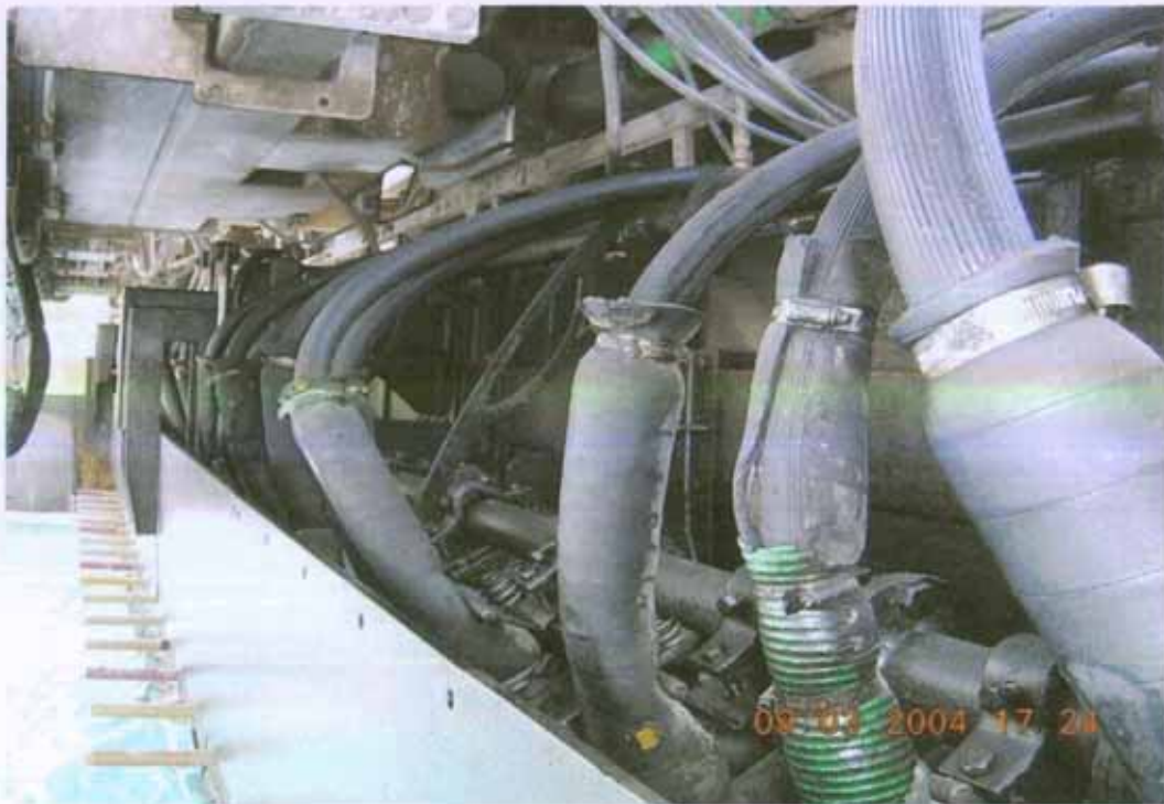
Vibrators Attached to Paver
