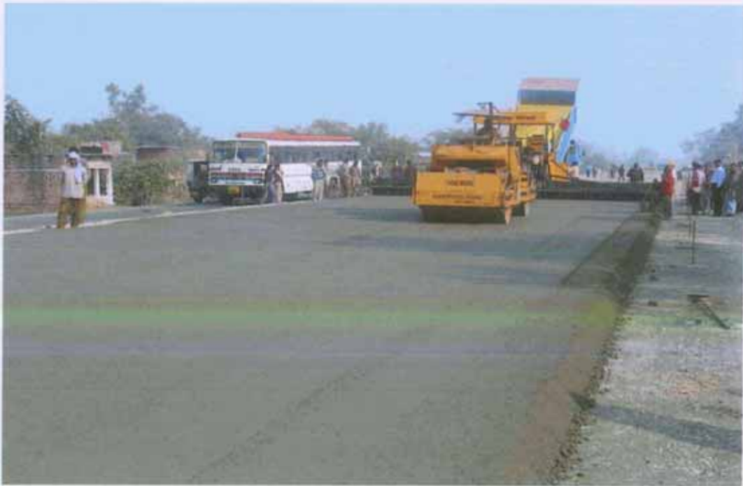
DLC laid and Compacted
