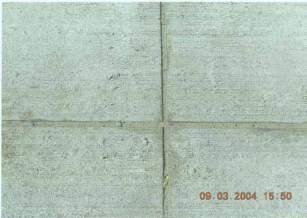
Proper Joint Cutting without Spalling
