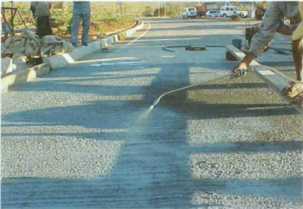
Curing compound on freshly laid concrete
