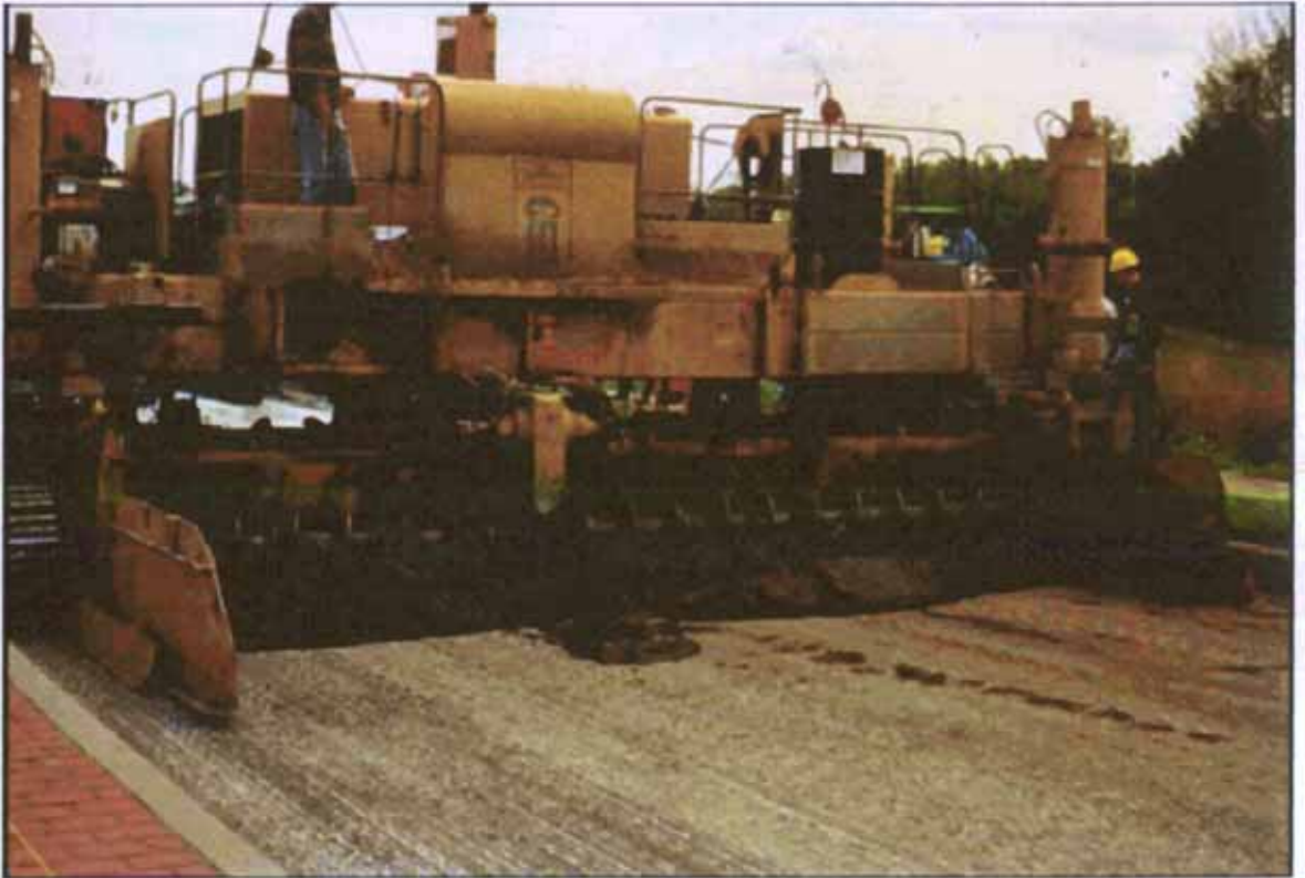
Placement using Slipform paver
