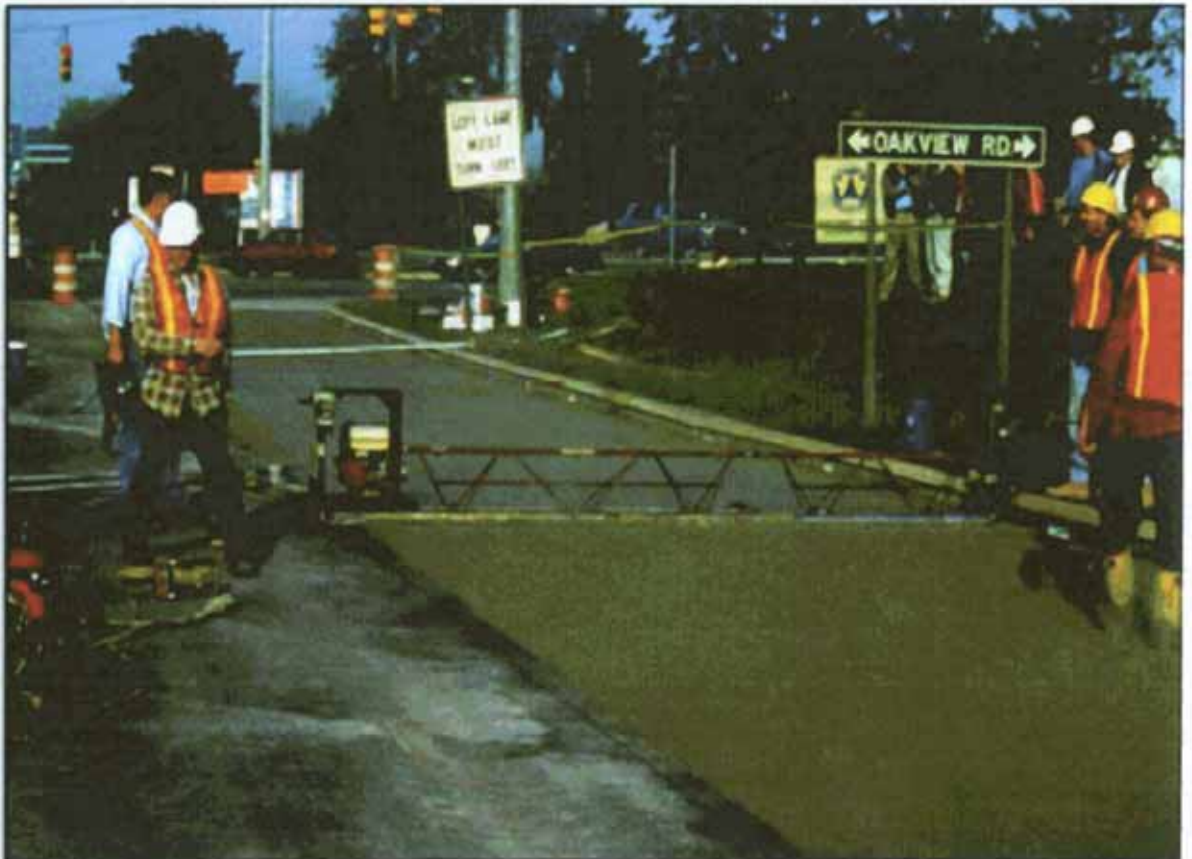
Placement using Vibrating Screed
