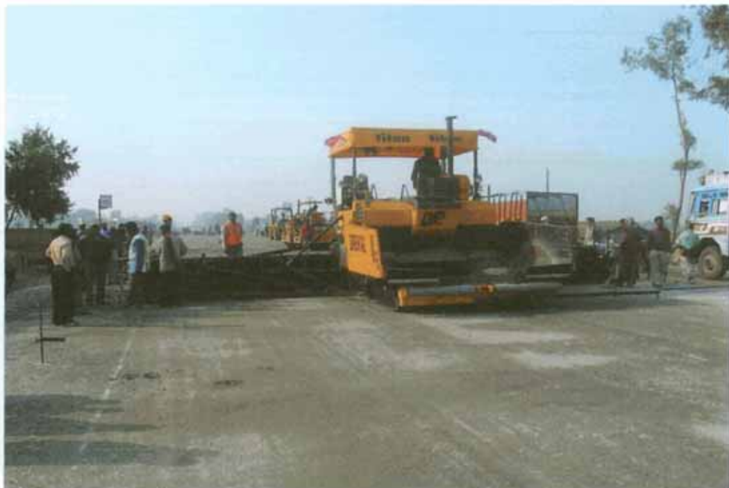
Dry Lean Concrete Paver
