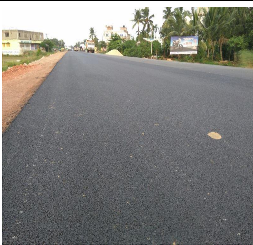
BC Laying at 33+760 to 34+600 LHS
