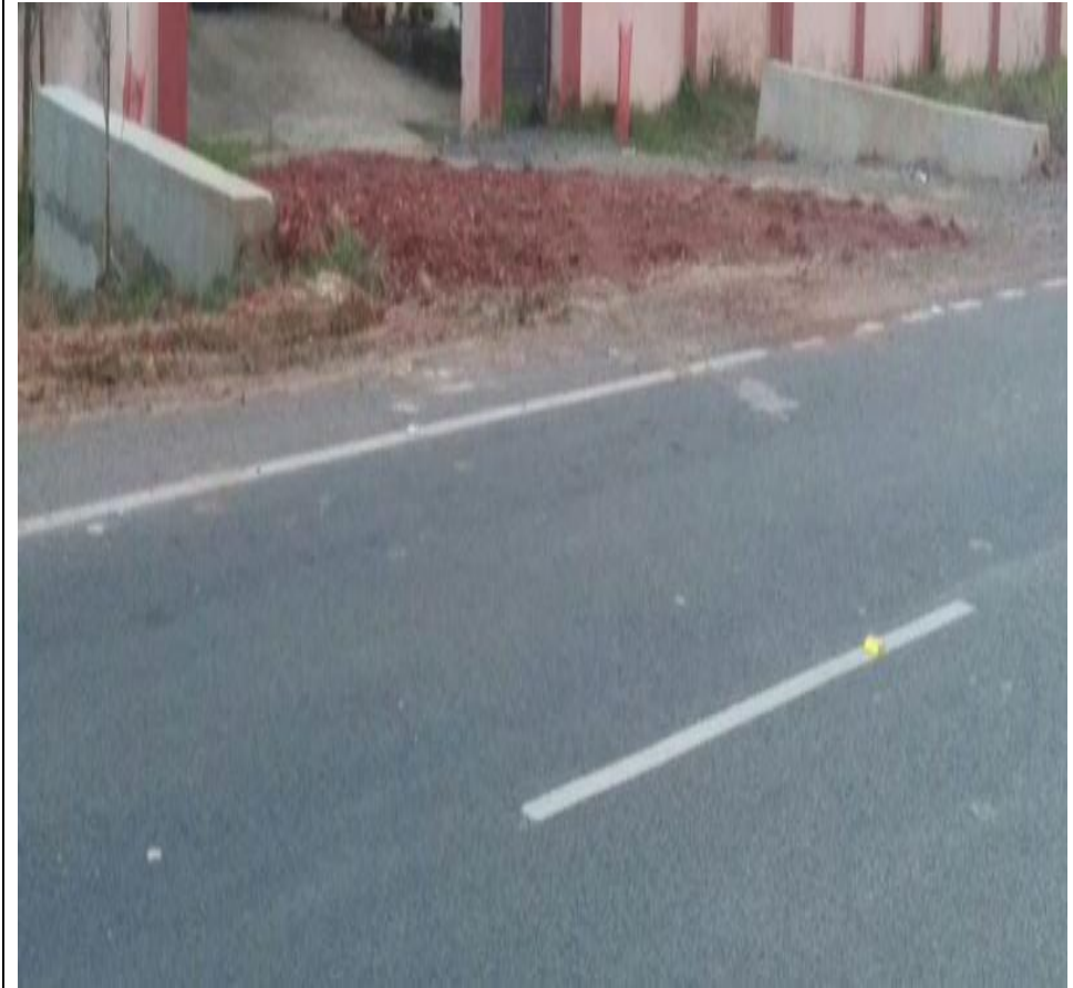
Access Road Culvert at 33+890 RHS
