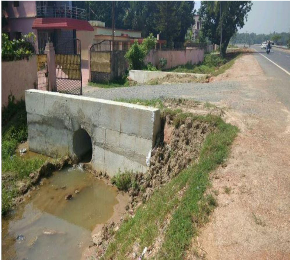
Access Road Culvert at 33+923 RHS
