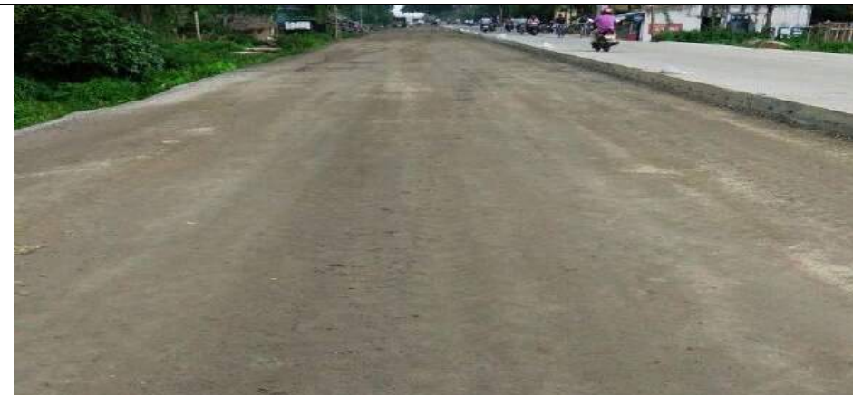
DLC laying from Ch. 53+800 to 54+000 (RHS)
