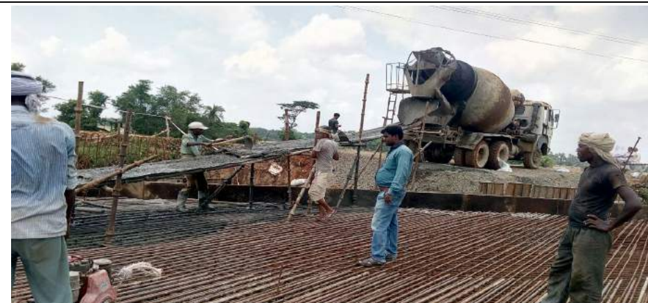
Slab Casting at Ch. 69+727
