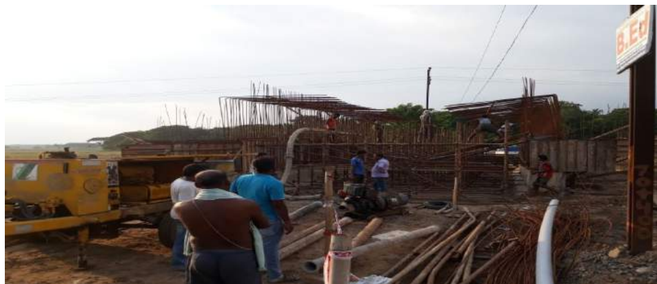
Concreting of PUP at Ch. 70+401 2 nd lift wall
