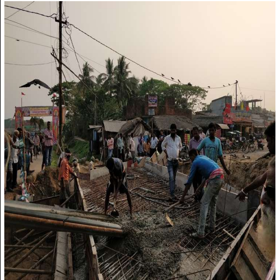
Box Culvert Deck Slab Concrete at 38+937 RHS
