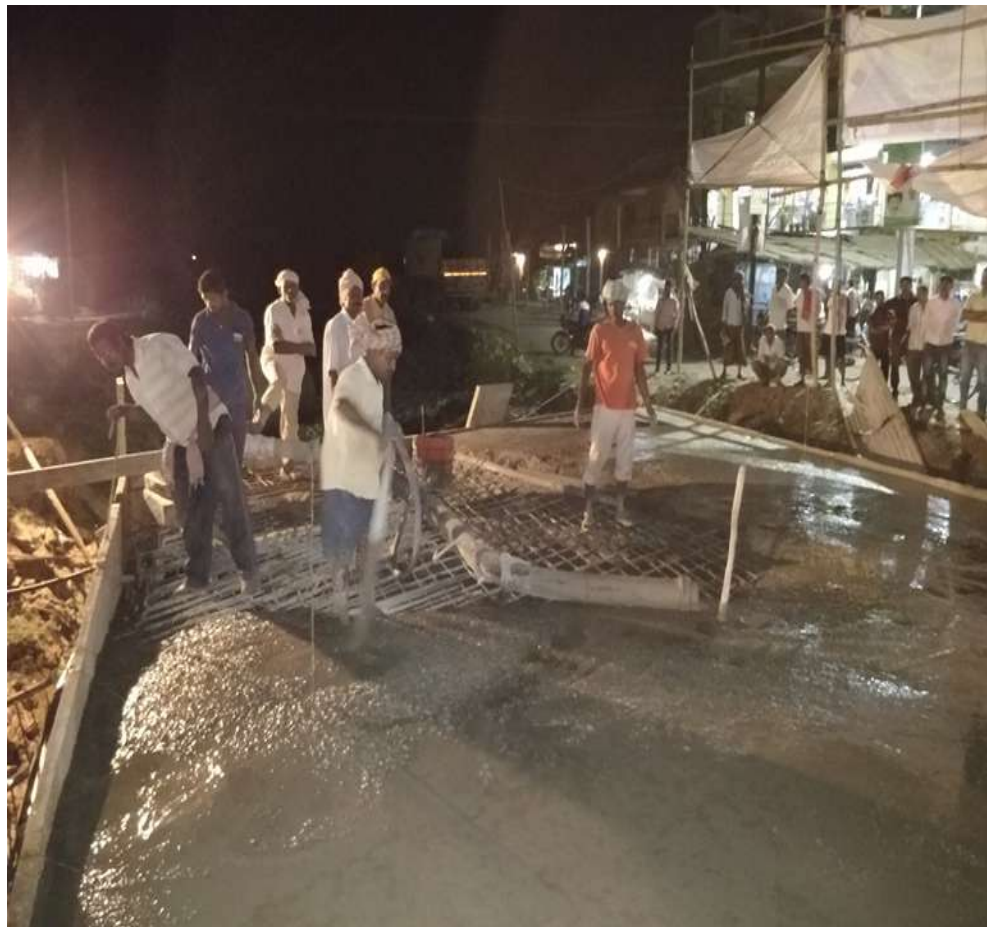
Box Culvert Deck Slab Concrete at 28+173 RHS
