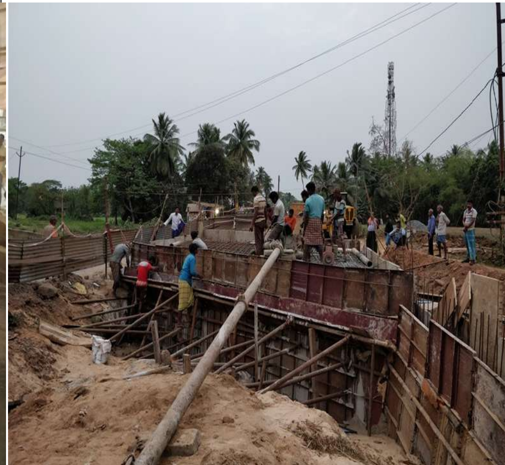
Box Culvert Deck Slab Concrete at 32+978 LHS
