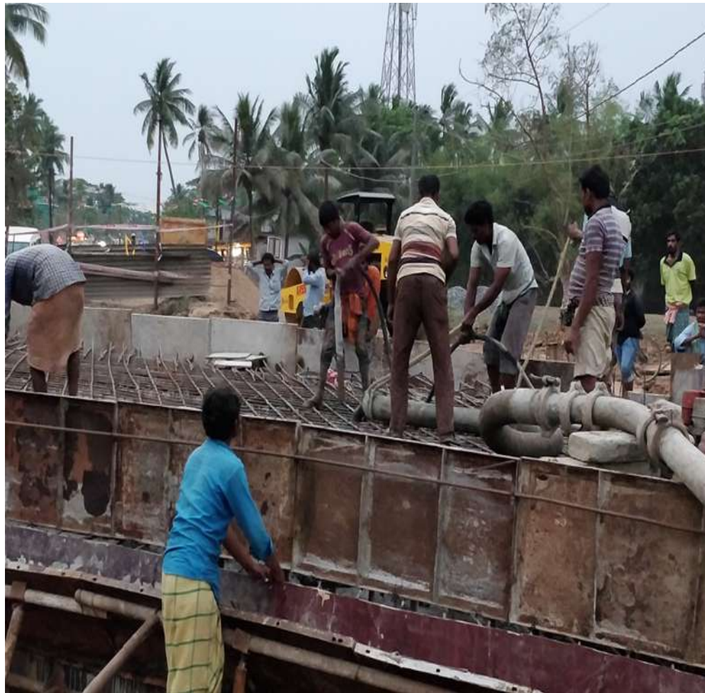
Box Culvert Deck Slab Concrete at 32+978 LHS
