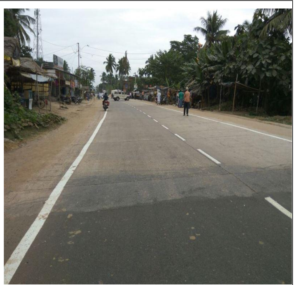
Road Marking at 32+030 to 32+650 RHS
