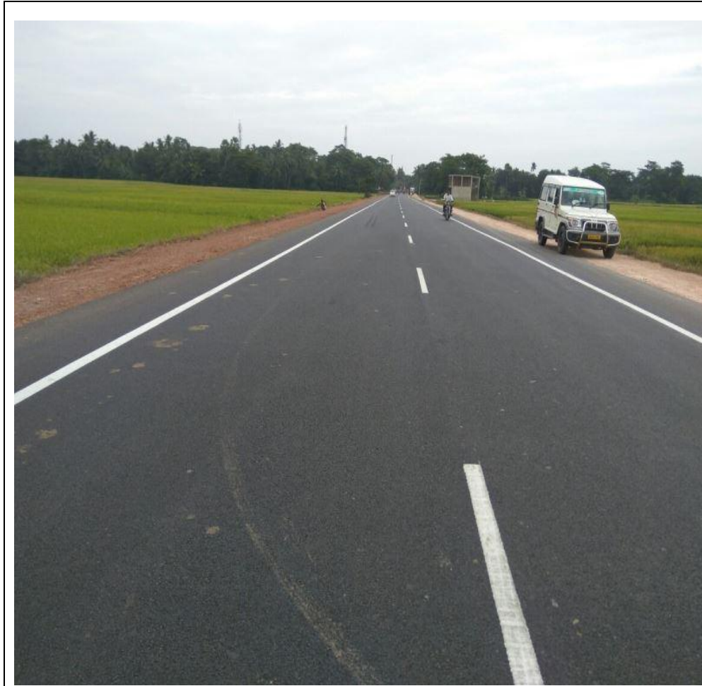
Road Marking at 28+400 to 29+189LHS
