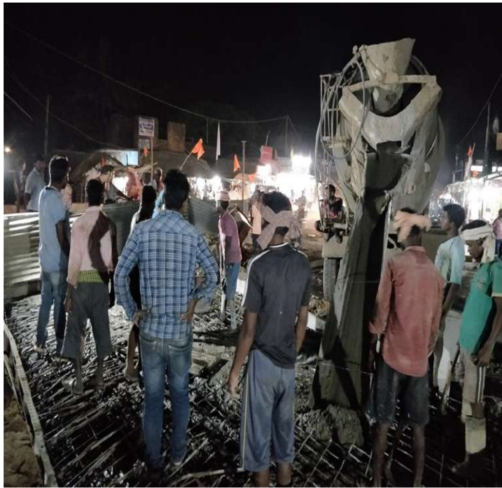
Box Culvert Deck Slab Concrete at 38+937 LHS
