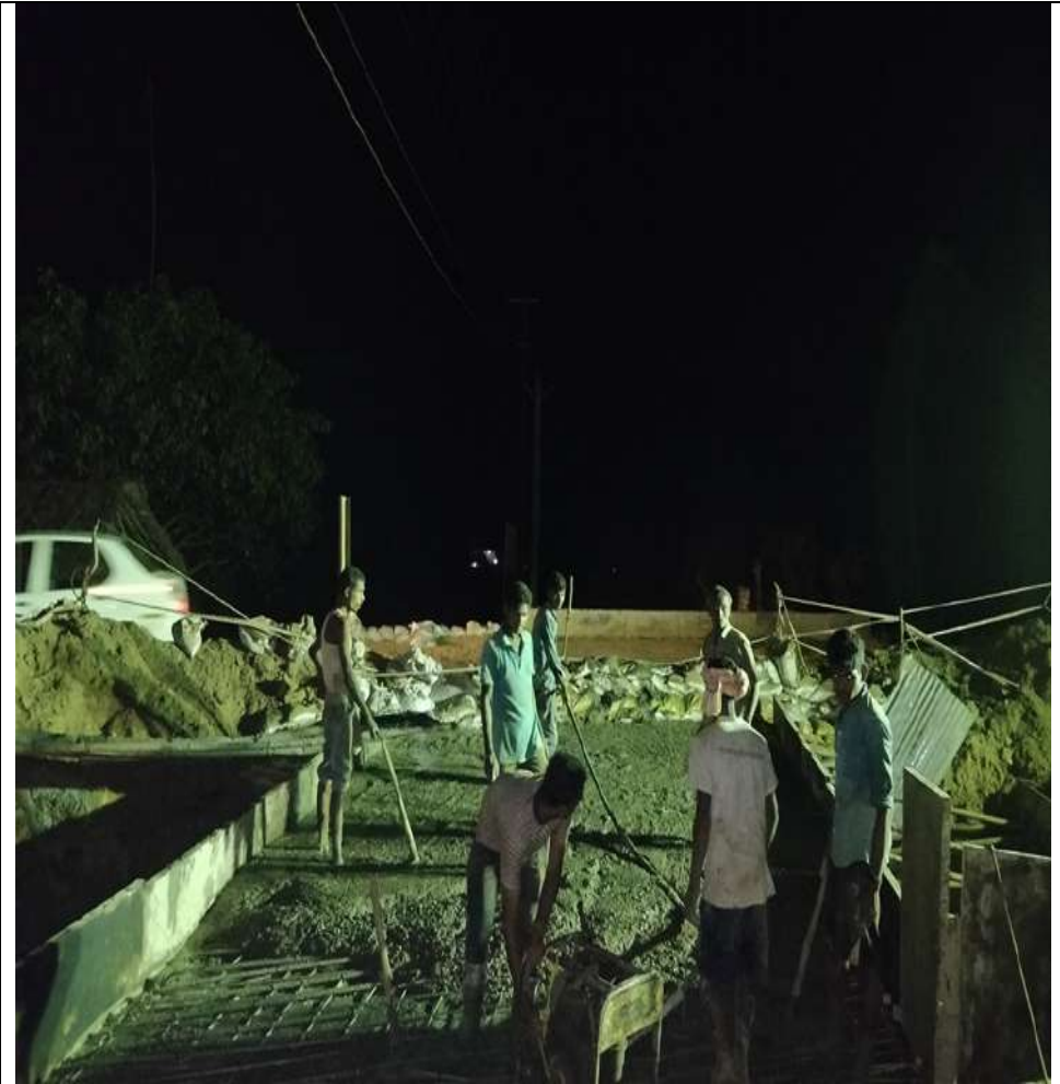
Box Culvert Deck Slab Concrete at 32+978 RHS
