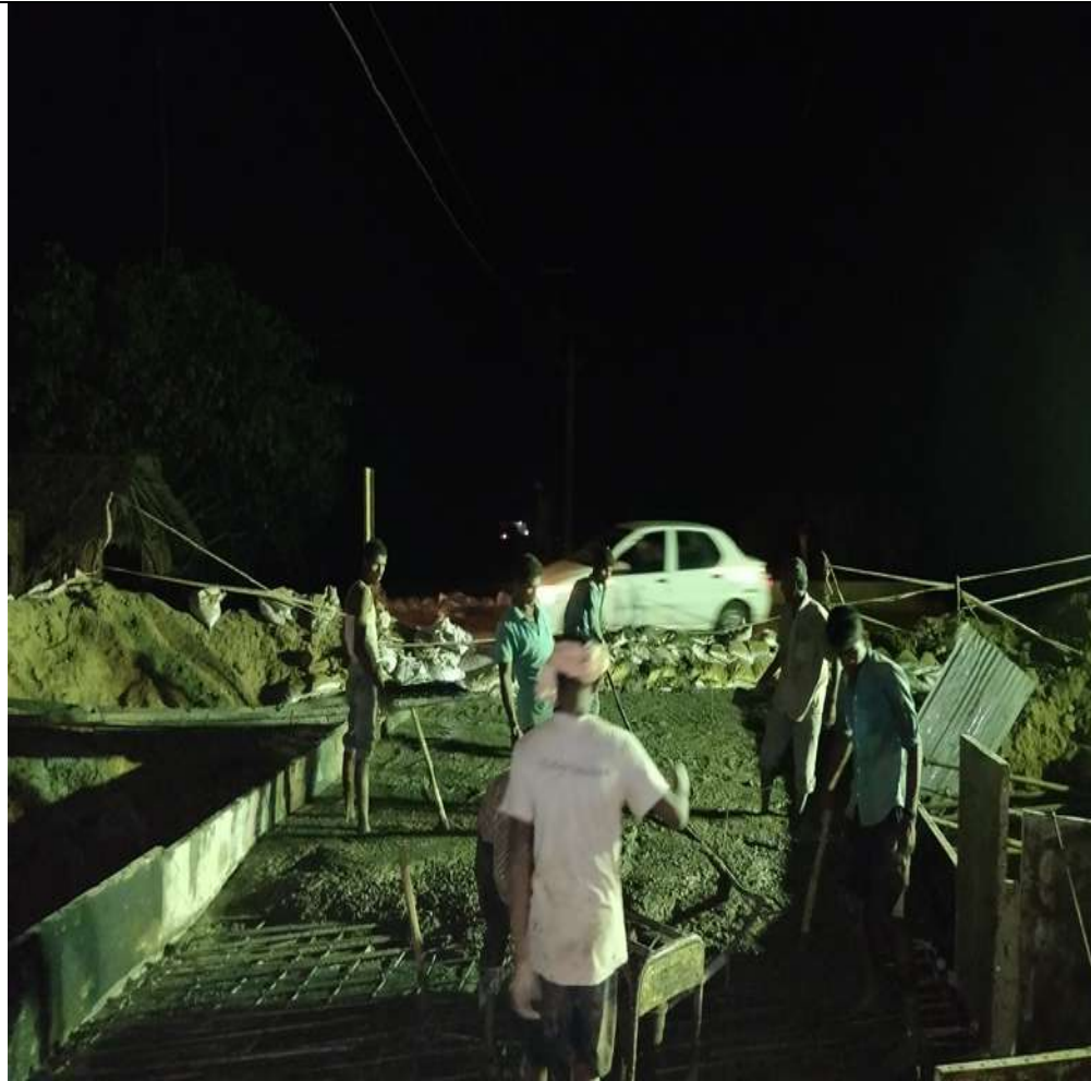
Box Culvert Deck Slab Concrete at 32+978RHS
