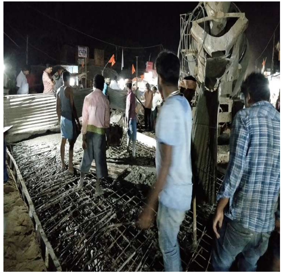
Box Culvert Deck Slab Concrete at 38+937 LHS
