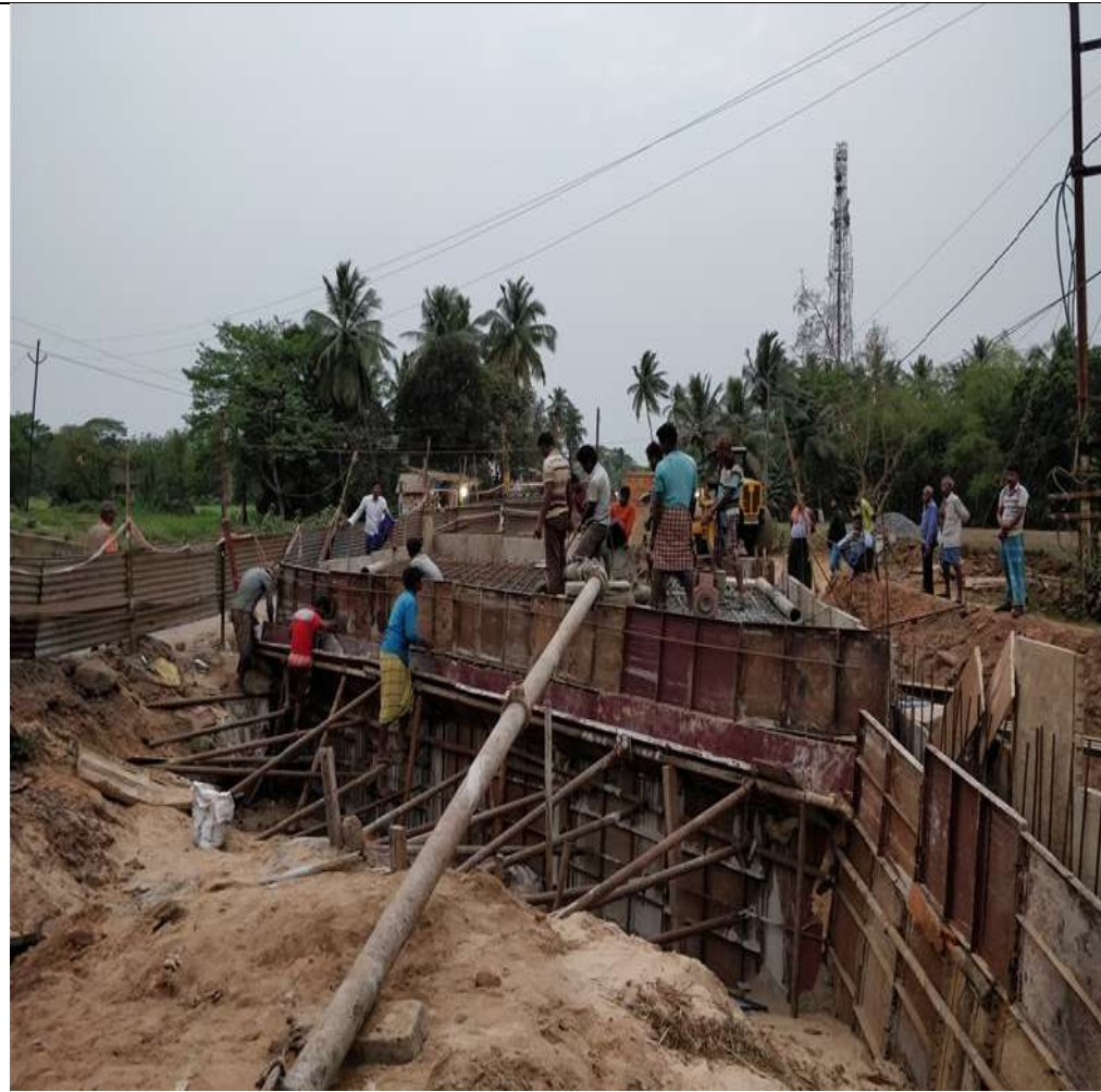
Box Culvert Deck Slab Concrete at 32+978LHS
