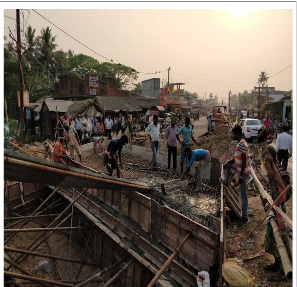
Box Culvert Deck Slab Concrete at 38+937 RHS
