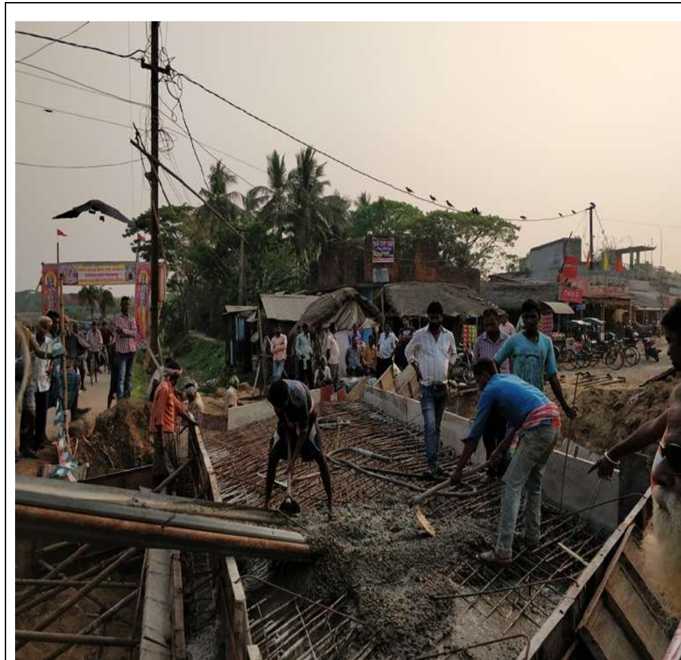
Box Culvert Deck Slab Concrete at 38+937 RHS
