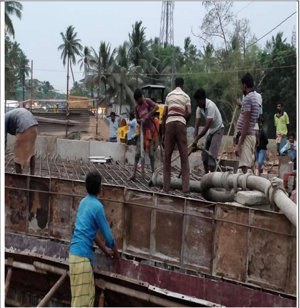
Box Culvert Deck Slab Concrete at 32+978 LHS
