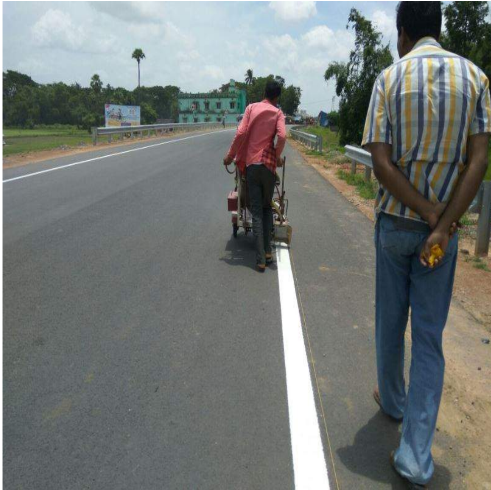
Road Marking at 44+022 to 44+300 Edge line RHS
