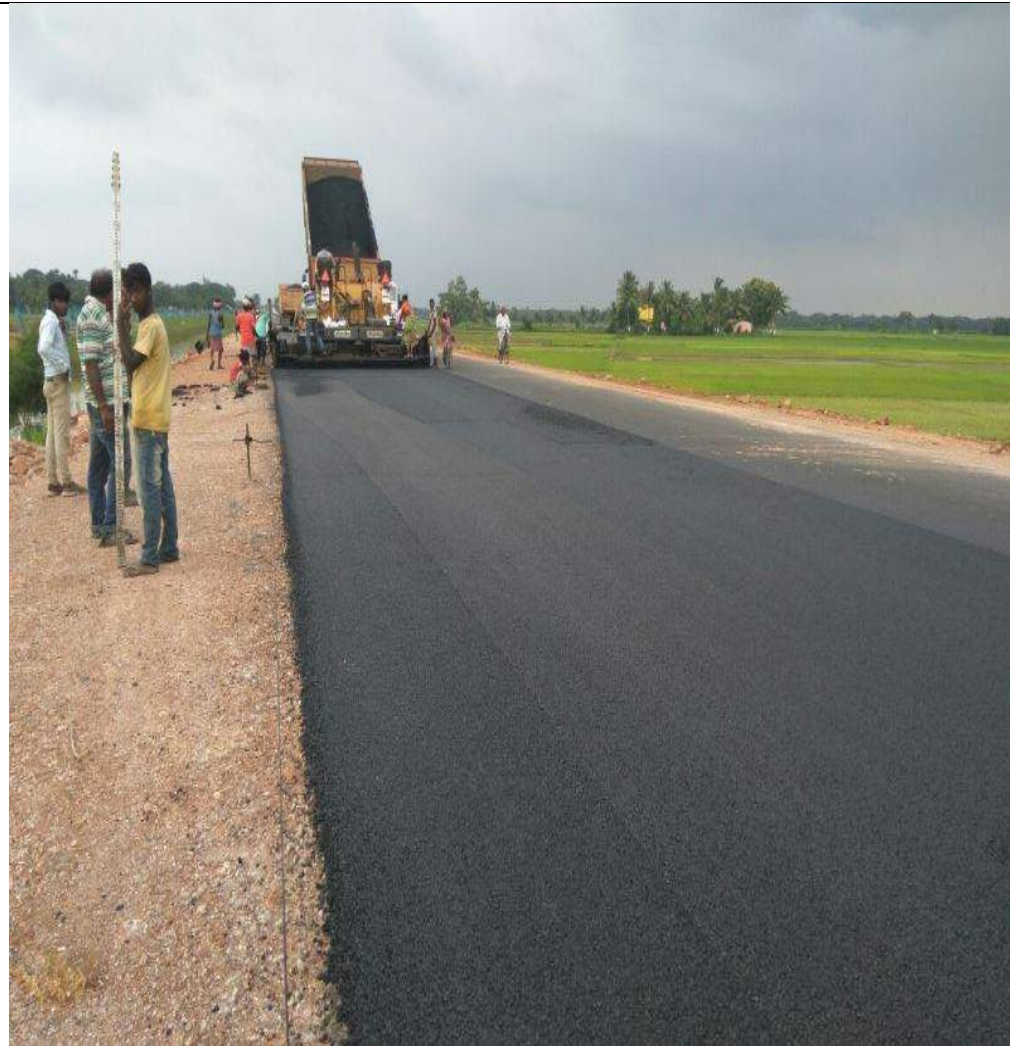
BC Laying at 31+300 to 32+040LHS
