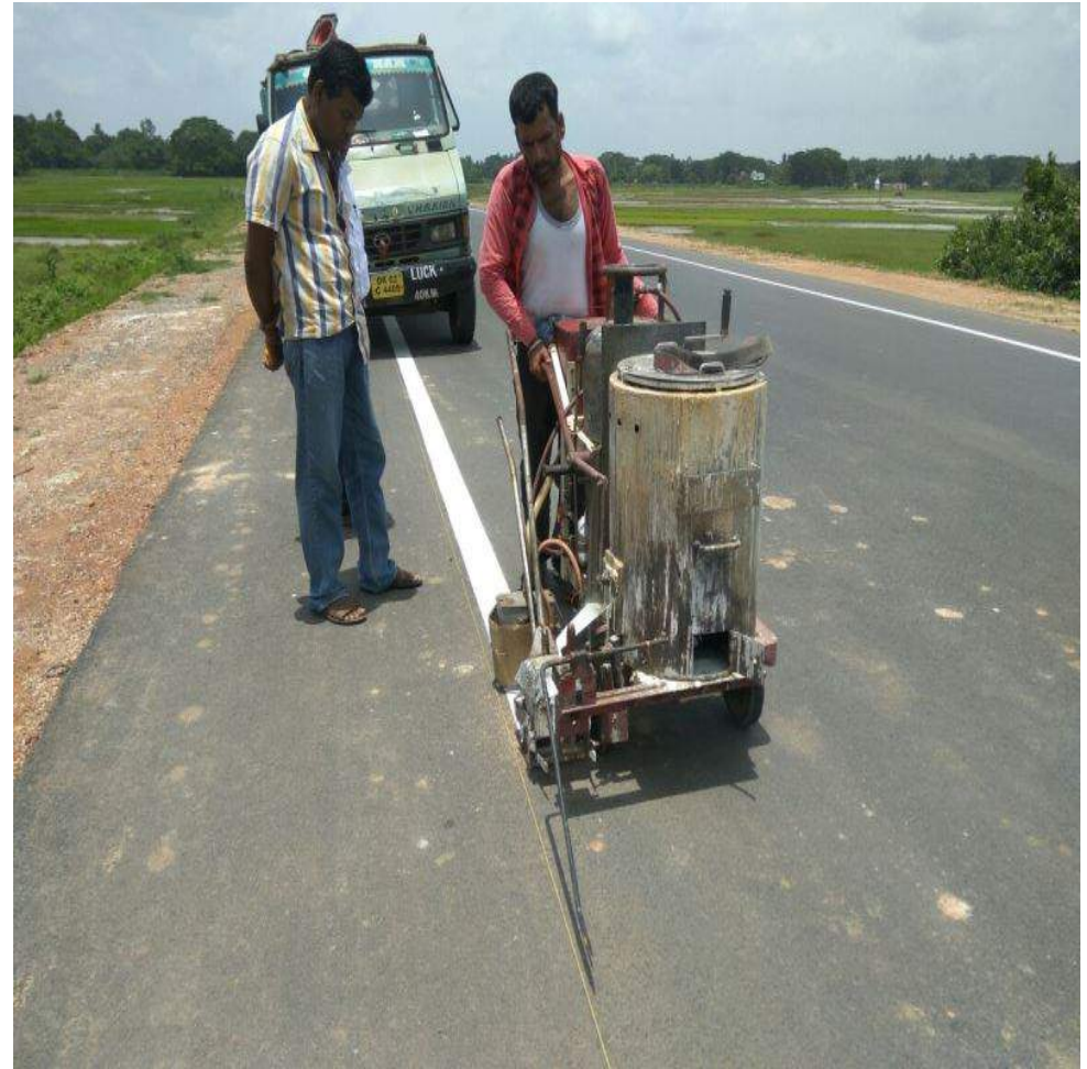
Road Marking at 33+200 to 34+200 Edge line LHS
