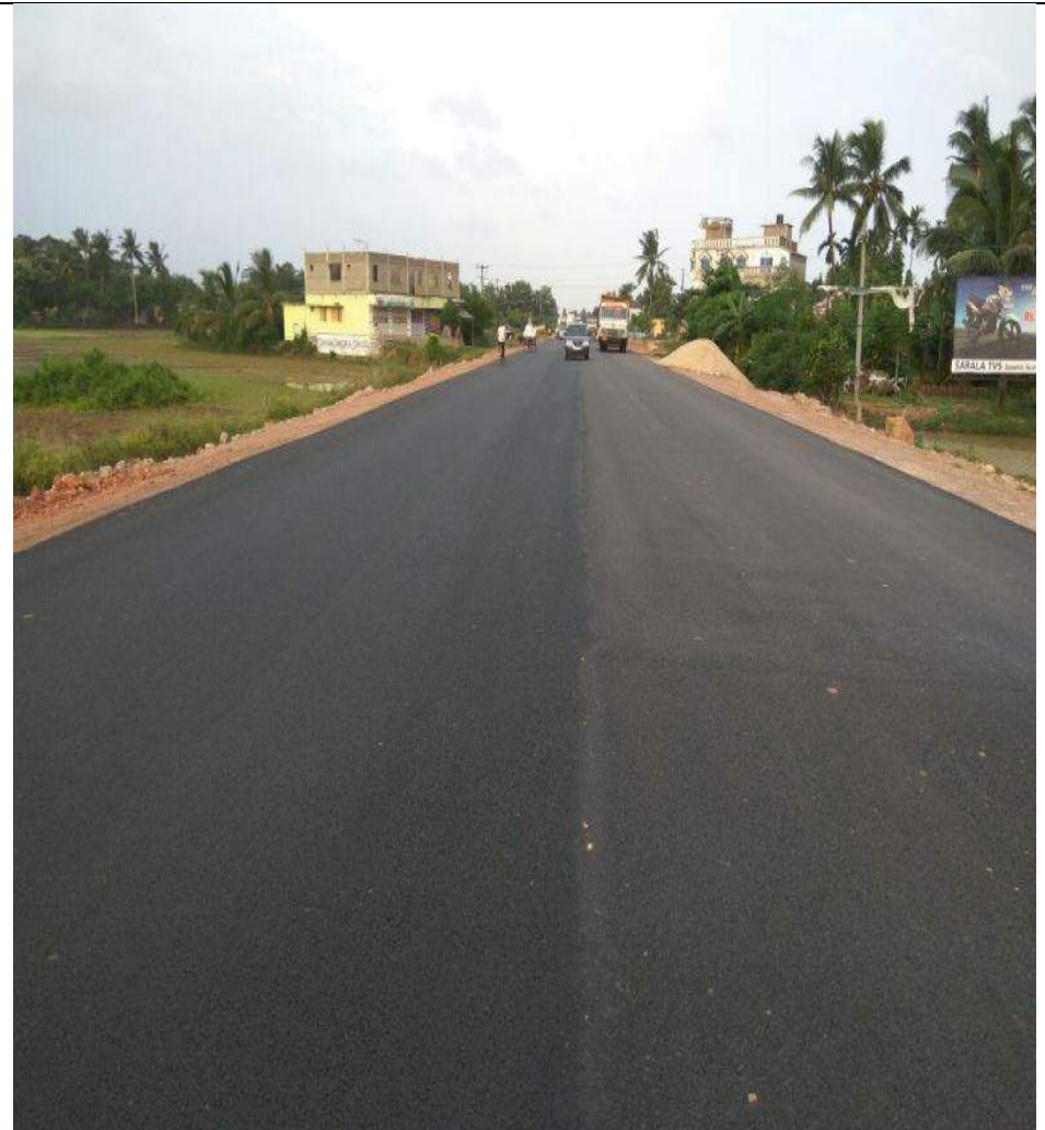
BC Laying at 25+000 to 25+360 RHS
