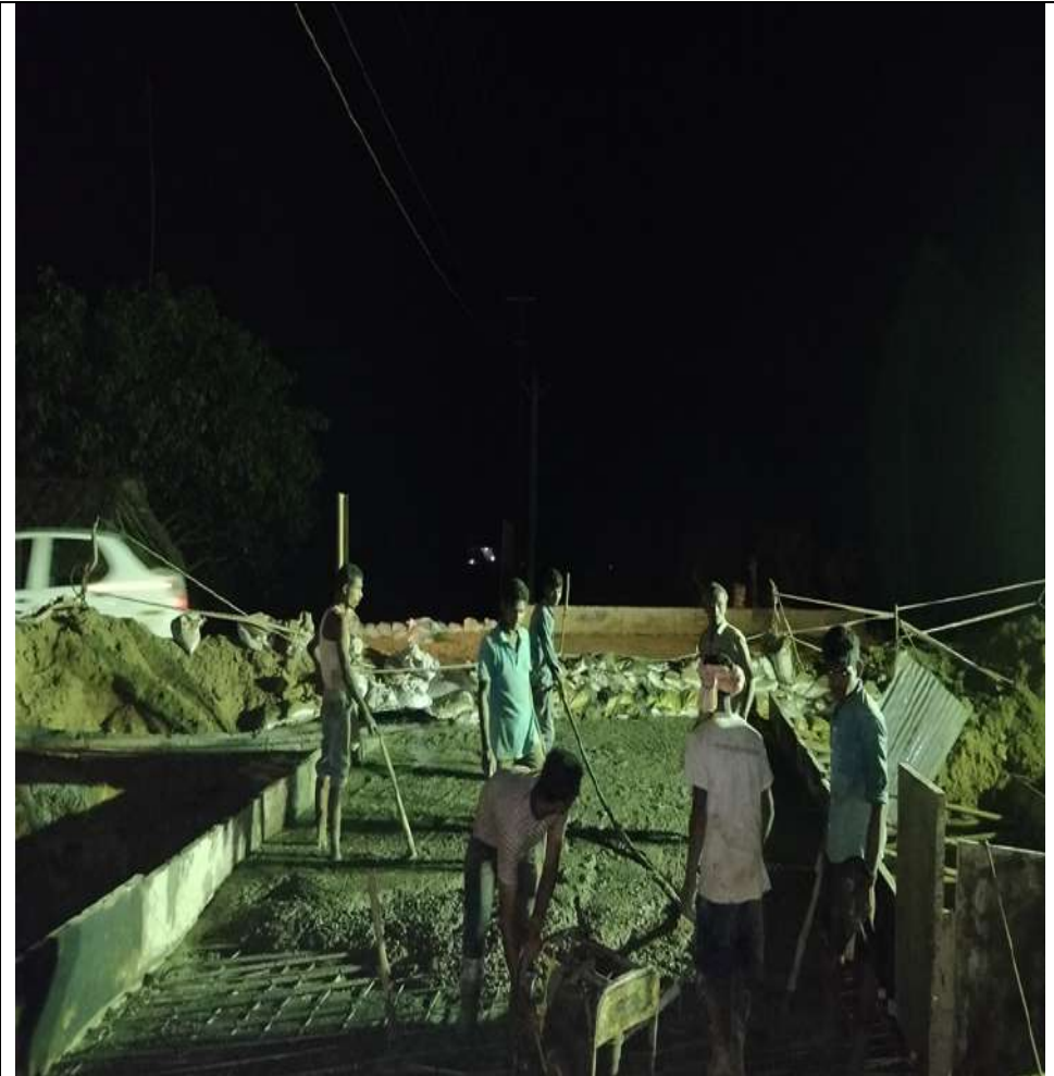
Box Culvert Deck Slab Concrete at 32+978 RHS
