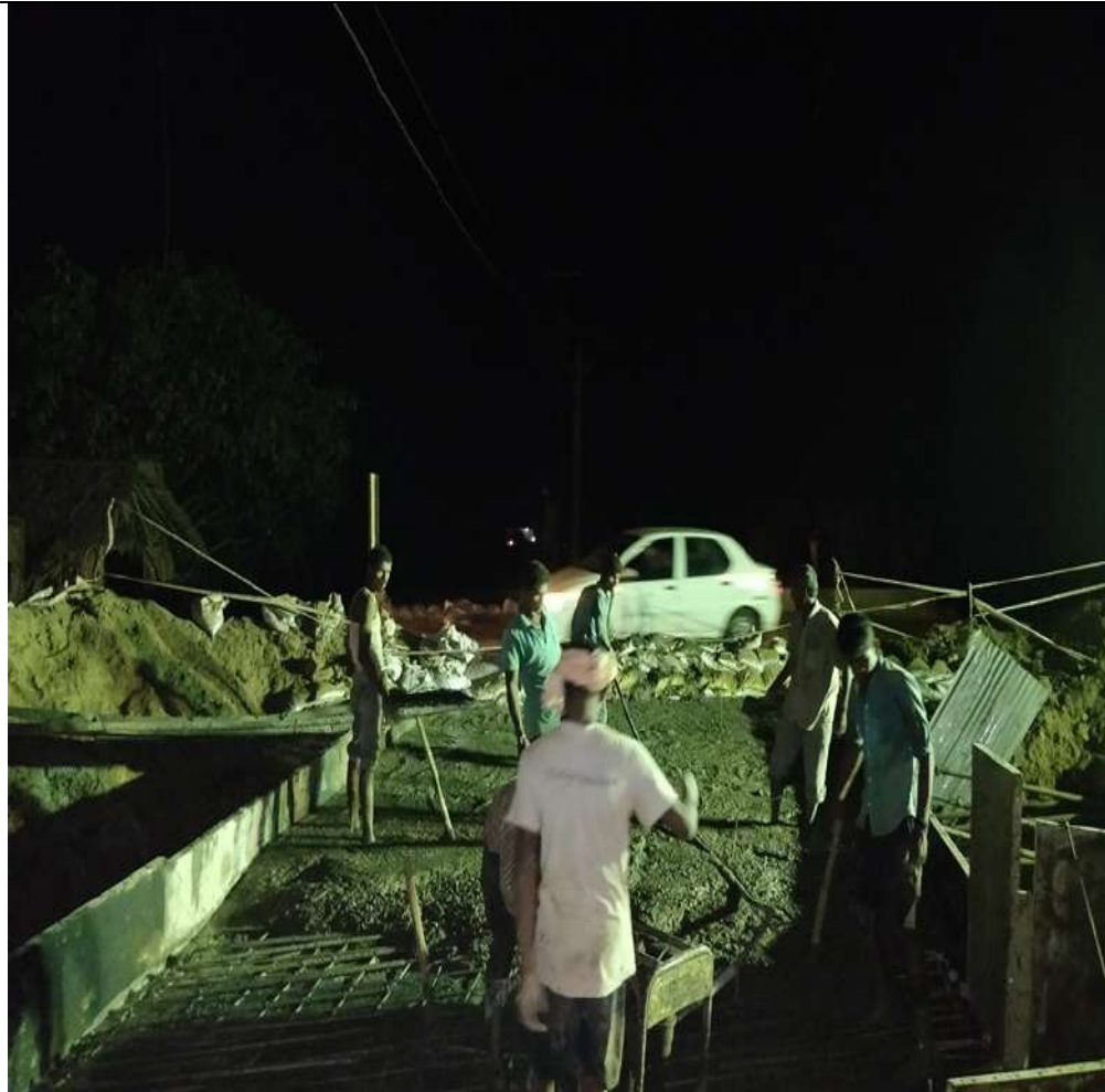
Box Culvert Deck Slab Concrete at 32+978RHS
