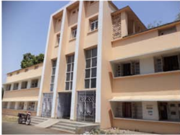
R&B & NH Sambalpur Division Office
